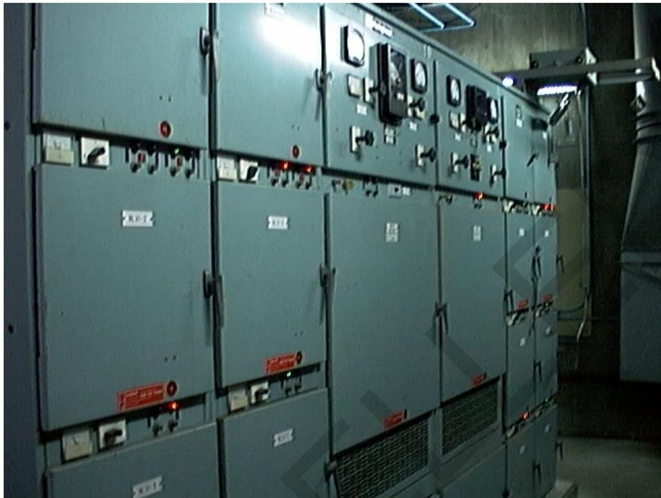
**Figure 13-4. Skid-Mounted Substation**
