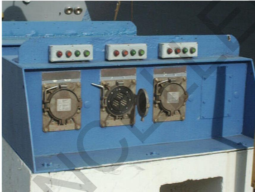
\2\ Figure 13-8. 4.16 kV Pier Electrical Outlet Assembly and Outlets – Existing Installations /2/
