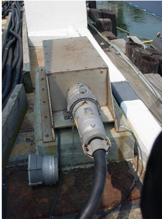
Figure 13-2. Close-Up of Electrical Connection Outlet Assembly
