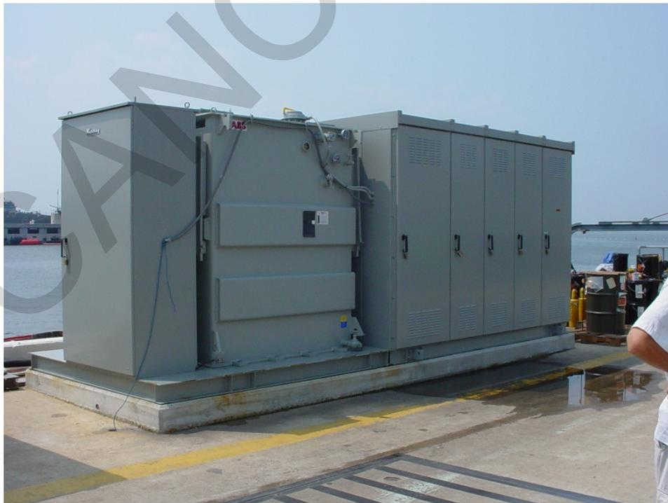
Figure 13-5. Skid-Mounted Substation with Single-Pole Connections
