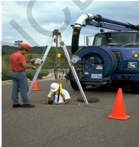
14-3.5 A tripod and retrieval system is the best method for both the victim and the rescuer. With this method one worker can perform the rescue, and even the smallest individuals can rescue a large victim.
