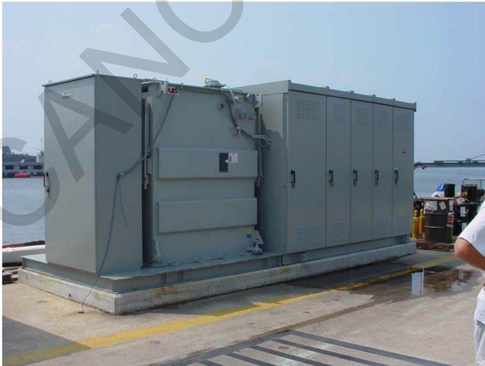
Figure 13-5. Skid-Mounted Substation with Single-Pole Connections
