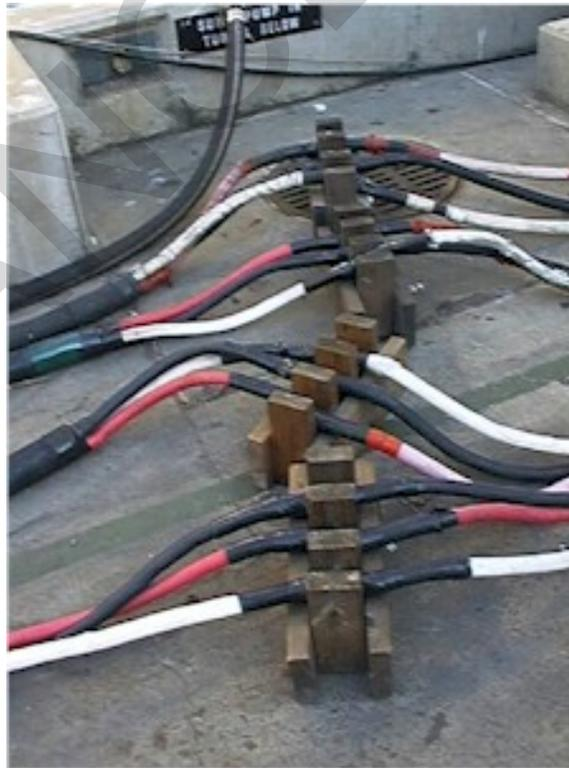
13-3 **SHIP'S ELECTRICAL SERVICE COMPONENT RELATIONS.** An understanding of the physical and electrical arrangements of these components is necessary in understanding the safety problems involved in the basics of using portable power cables to feed shore electrical power to a ship's electrical bus.
