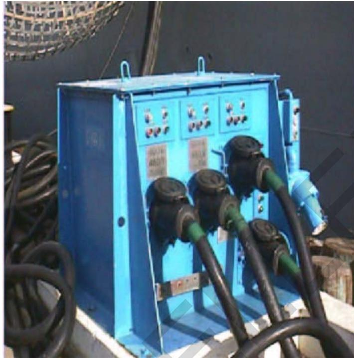
Figure 13-11. 480 Volt Shore-Cable to Ship-Cable with Single-Pole Connection
