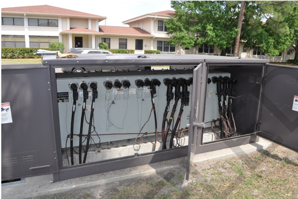
Figure D-2 G&W VFI Switchgear
