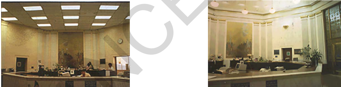
Figure B-6. Example of the same space with downlighting only (left) and then with improved surface brightness (right)
