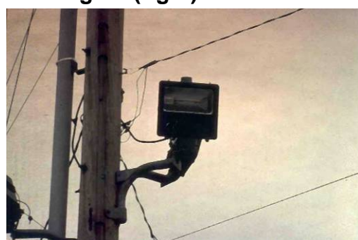
Figure D-5. Fully shielded or IES fully shielded luminaires (left) are recommended. Do not use unshielded floodlights (right)
