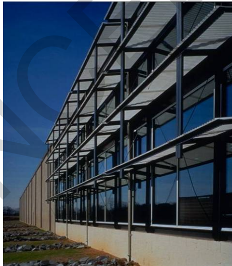
Figure 4-4. Example of architectural shading devices.
