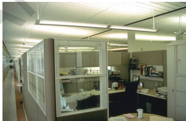
Figure 2-4. Semi-indirect lighting minimizes indirect glare.
