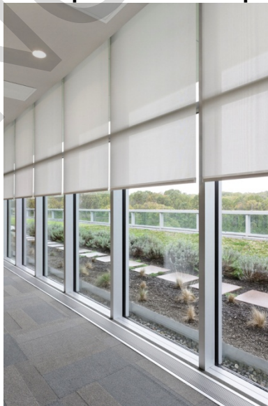
Figure 4-12 Example of Solar-Adaptive Shading
