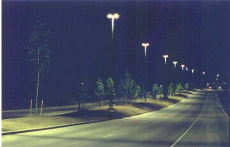
Figure 3-3. Examples of IES \2\ fully shielded /2/ luminaires.
