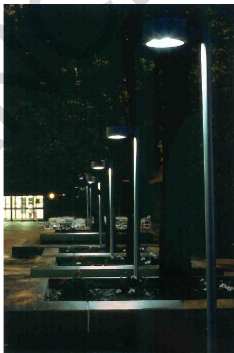
Figure 2-2. Minimize direct glare with IES \2\ fully shielded /2/ luminaire.
