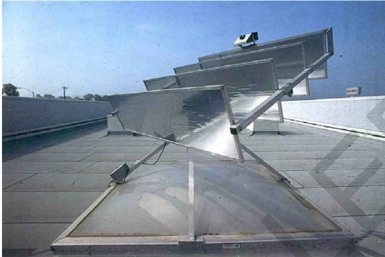
Figure 4-11. Example of an Active Daylighting System that Tracks the Sun and Directs Daylight into the Building.
