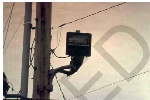
Figure 3-5. Fully shielded or IES \2\ fully shielded /2/ luminaires (left) are recommended. Do not use unshielded floodlights (right).
