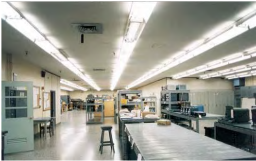
Figure 2-1. Examples of direct glare.
