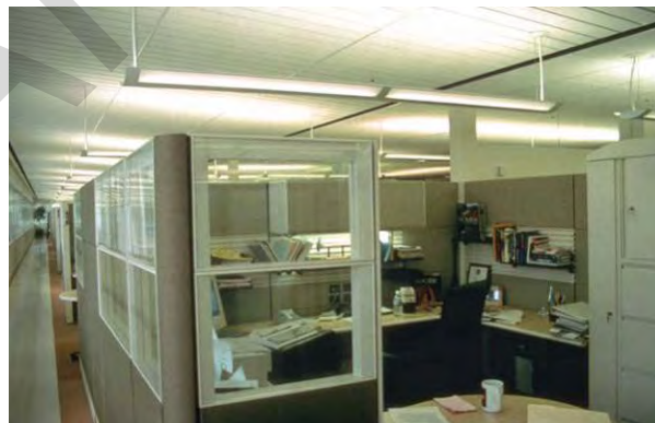
Figure 2-4. Semi-indirect lighting minimizes indirect glare.
