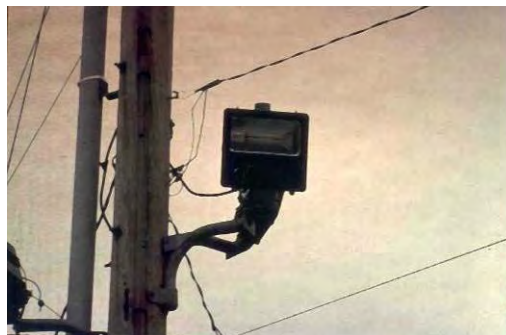
Figure 3-5. Fully shielded or IESNA full cut-off luminaires (left) are recommended. Do not use unshielded floodlights (right).
