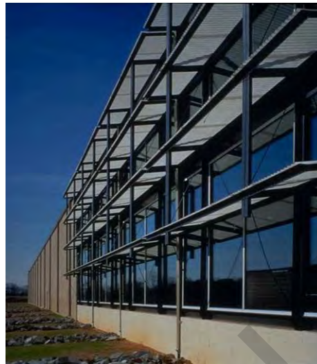
Figure 4-3. Example of architectural shading devices.
