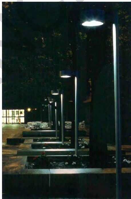
Figure 2-2. Minimize direct glare with IESNA full cut-off luminaire.
