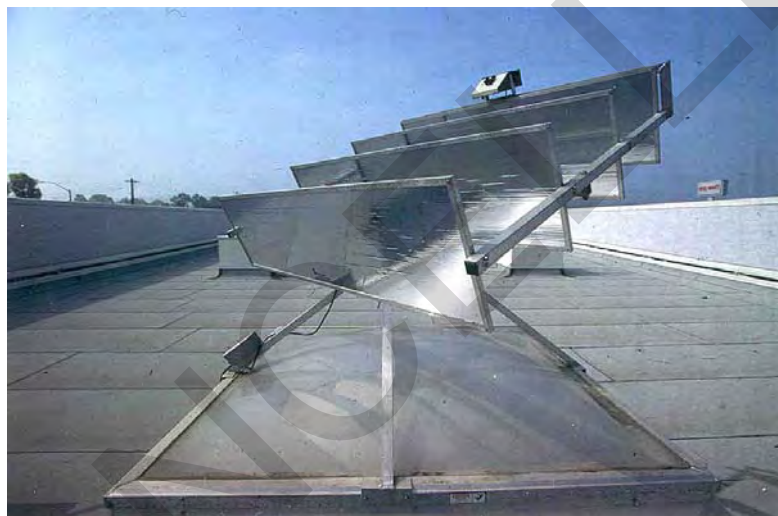
Figure 4-10. Example of an active daylighting system that tracks the sun and directs daylight into the building.
