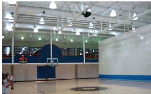
Figure 2-2. Minimize direct glare with IESNA full cut-off luminaire.
