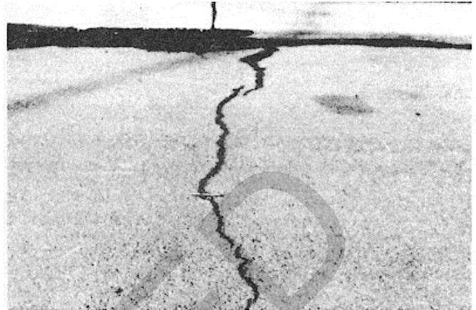
Figure B-39. Medium-severity longitudinal and transverse cracking.
