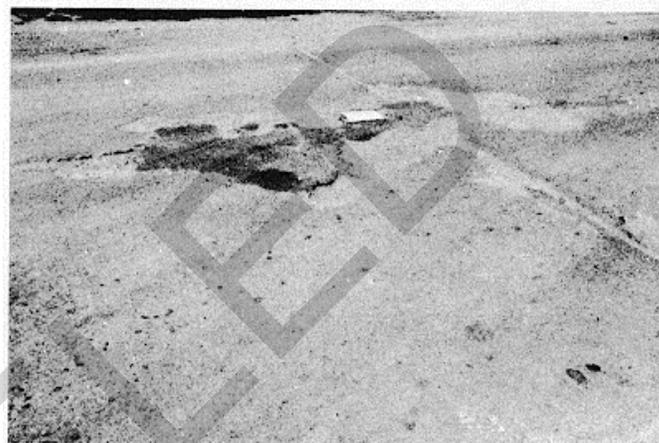
Figure B-129. High-severity scaling/map cracking/crazing.
