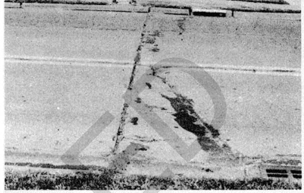
Figure B-121. Medium-severity punchout.
