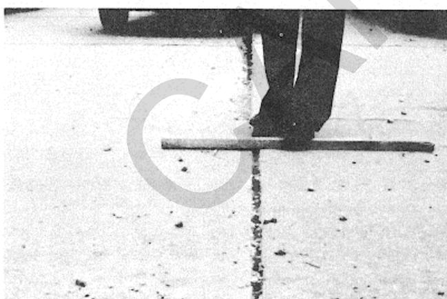
Figure B-90. Low-severity faulting.
