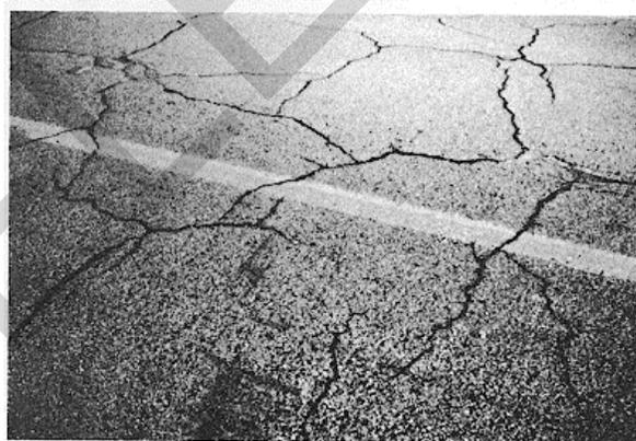
*Figure B-13. Medium-severity block cracking.*
