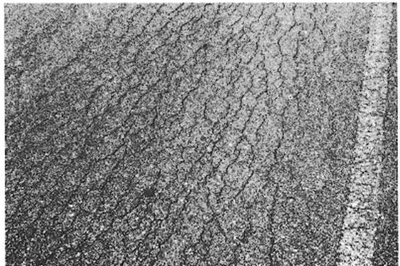
Figure B-5. Medium-severity alligator cracking.
