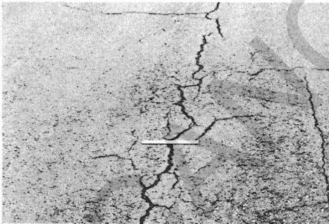
Figure B-40. Medium-severity longitudinal and transverse cracking (A  $\frac{1}{4}$  inch crack surrounded by light random cracks).
