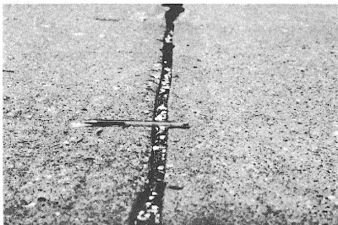
Figure B-96. High-severity joint seal damage.
