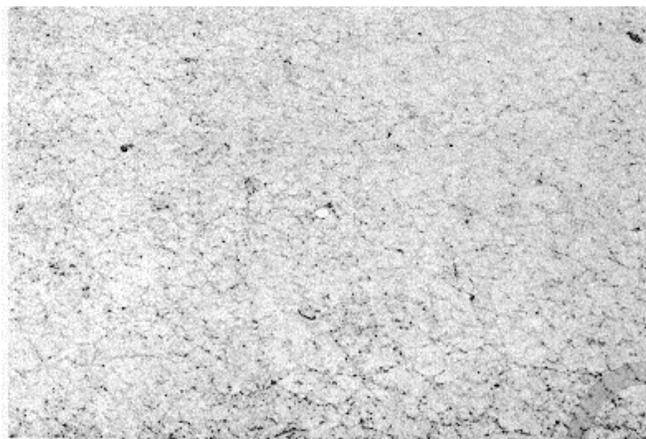
Figure B-126. Low-severity scaling/map cracking/crazing.
