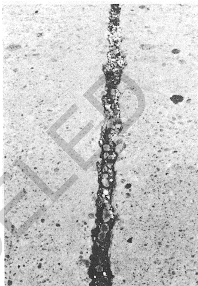
Figure B-97. High-severity joint seal damage.
