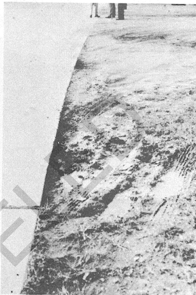
Figure B-99. Medium-severity lane/shoulder drop off
