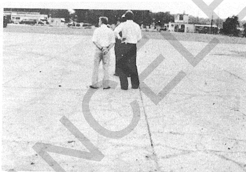
Figure B-84. High-severity divided slab.
