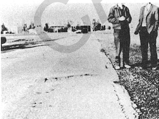
Figure B-16. Medium-severity bumps and sags.
