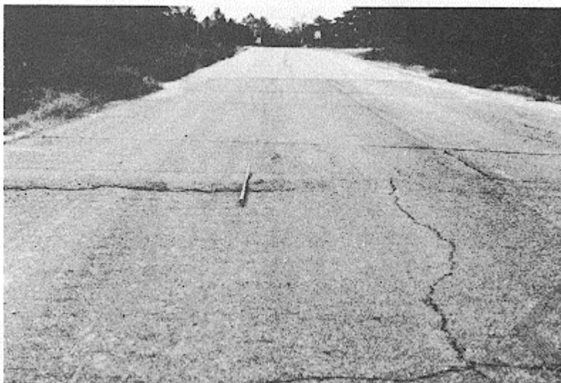
Figure B-18. Medium-severity bumps and sags.
