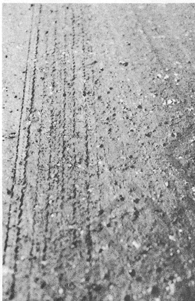
Figure B-10. High-severity bleeding.
