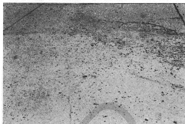
Figure B-89. High-severity durability cracking.
