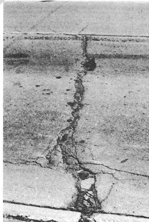
Figure B-41. High-severity longitudinal and transverse cracking.
