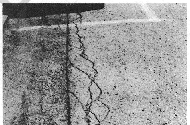
Figure B-28. Medium-severity edge cracking.
