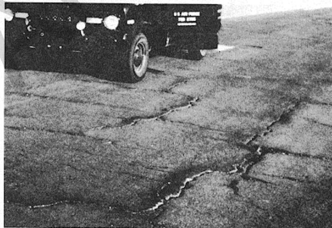
*Figure B-14. High-severity block cracking.*
