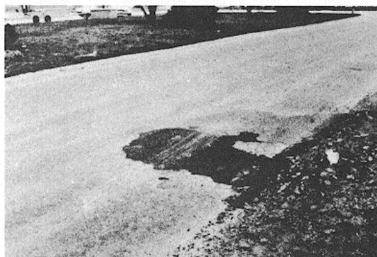
Figure B-45. Medium-severity patch.
