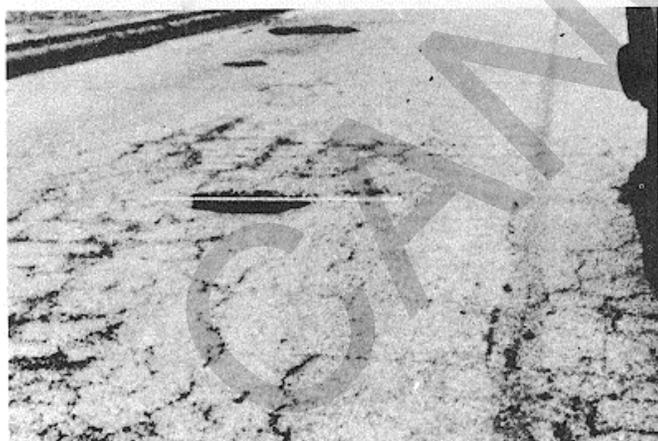
Figure B-50. Medium-severity pothole.
