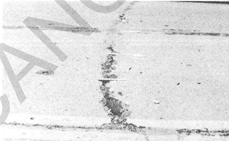
*Figure B-105. High-severity linear cracking in a nonreinforced concrete slab.*
