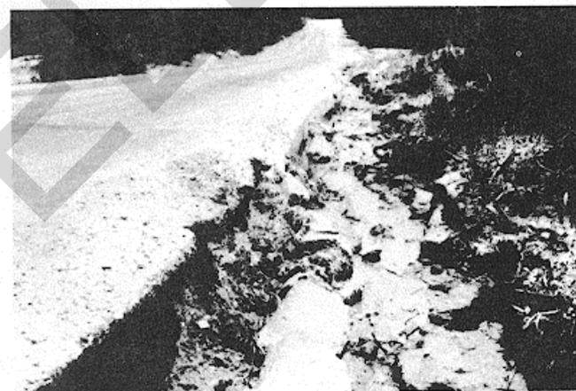
Figure B-37. High-severity lane/shoulder drop off
