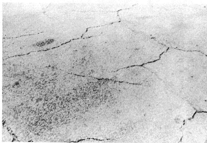
*Figure B-11. Low-severity block cracking.*
