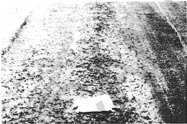
Figure B-69. Medium-severity weathering and raveling.
