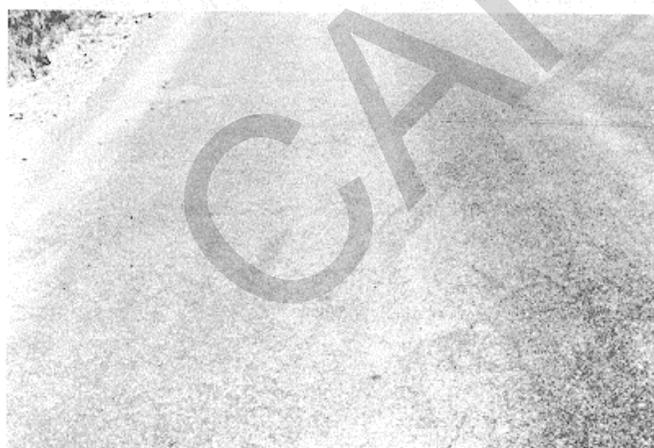
Figure B-8. Low-severity bleeding.
