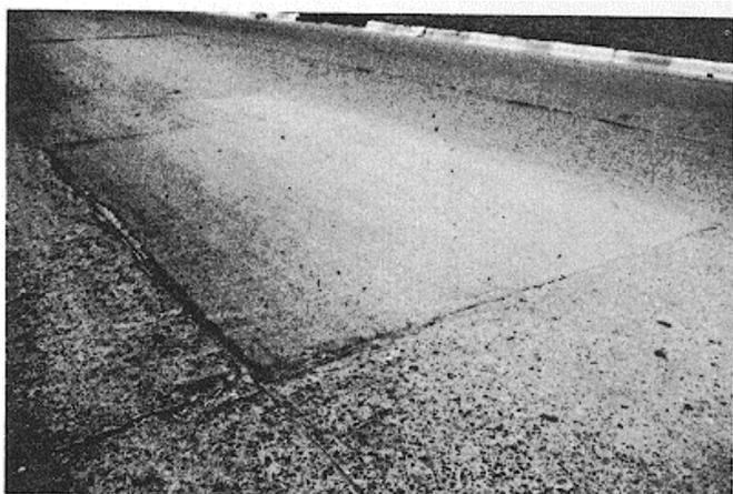
Figure B-107. Low-severity patching, large, and utility cuts.
