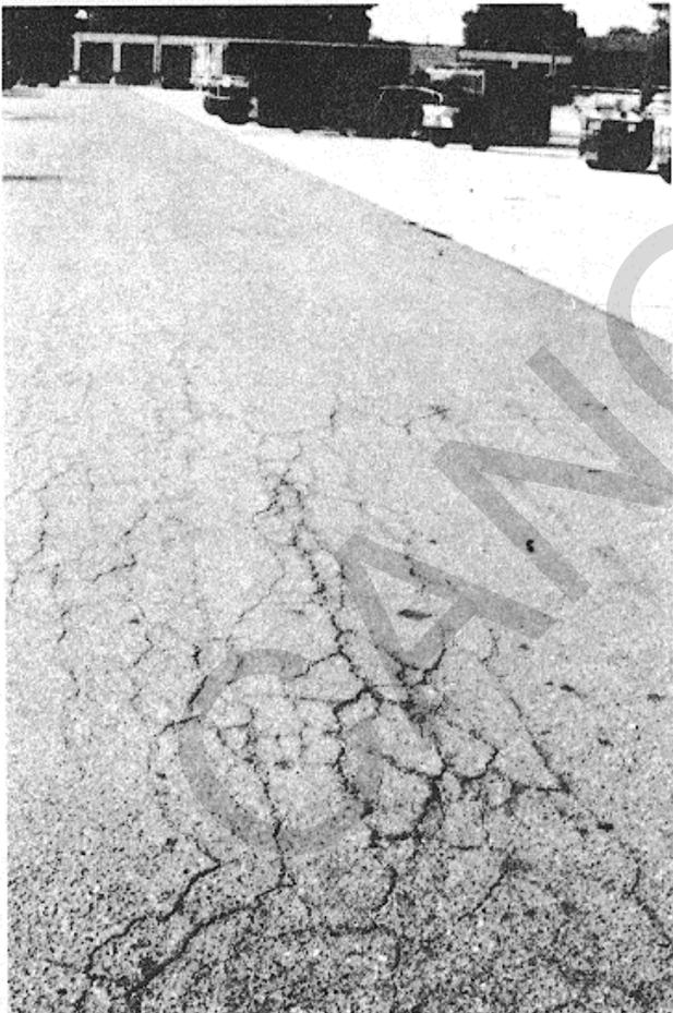
Figure B-3. Medium-severity alligator cracking
