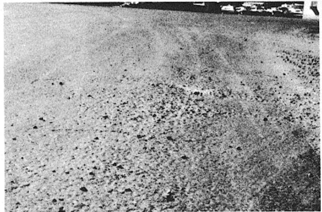
Figure B-70. Medium-severity weathering and raveling.
