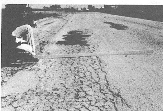
Figure B-6. High-severity alligator cracking.
