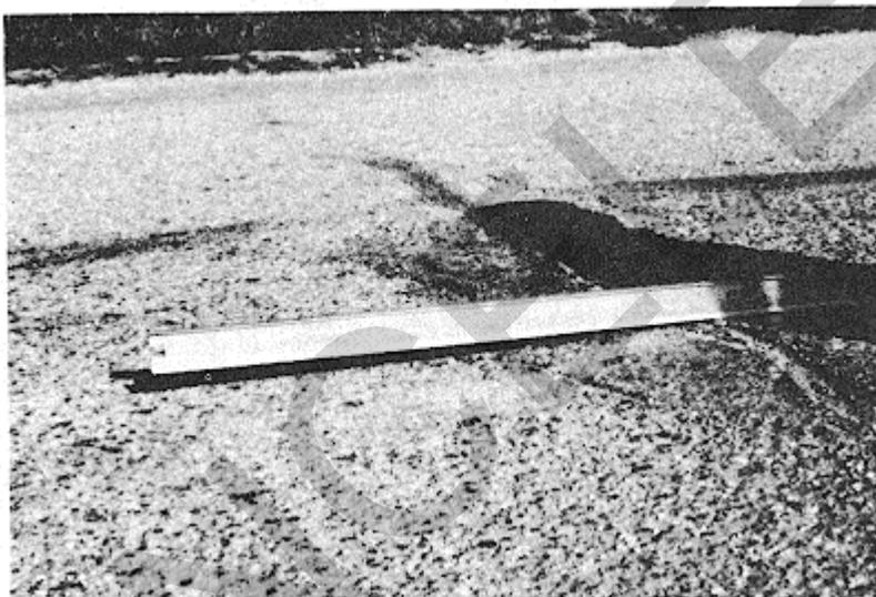
Figure B-15. Low-severity bumps and sags.
