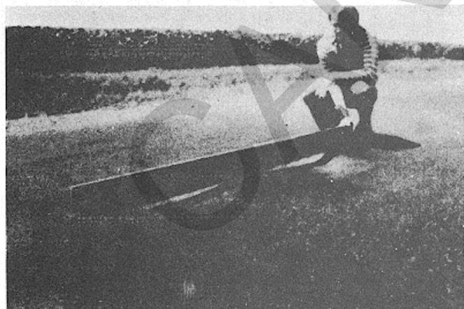
Figure B-23. High-severity corrugation.
