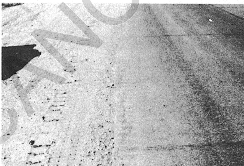
Figure B-31. Low-severity joint reflection cracking.
