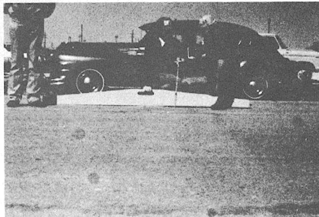
Figure B-24. Low-severity depression.
