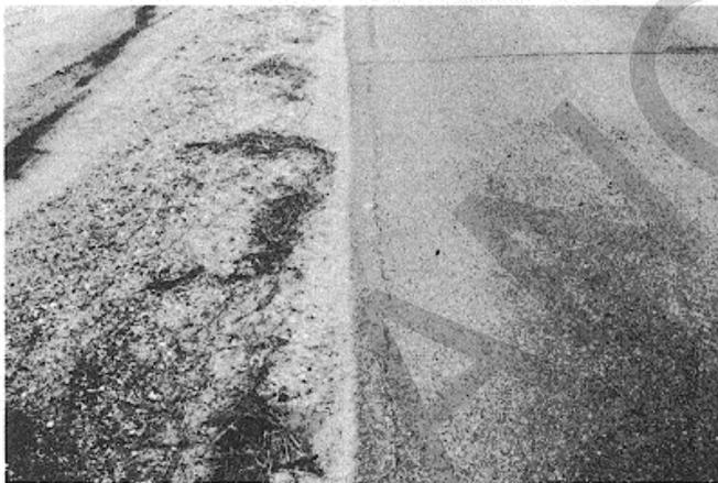
Figure B-27. Low-severity edge cracking.
