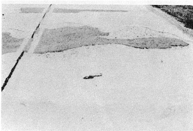
Figure B-128. High-severity scaling/map cracking/crazing.
