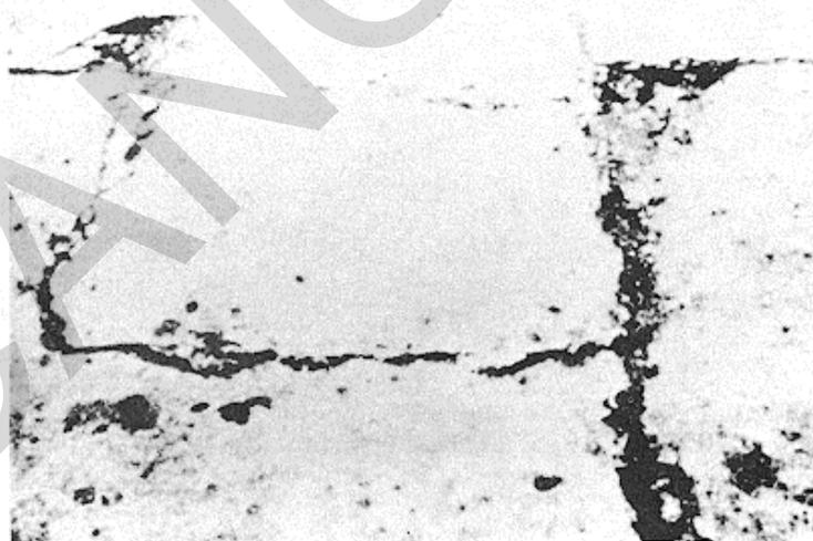
Figure B-112. High-severity patching, large.
