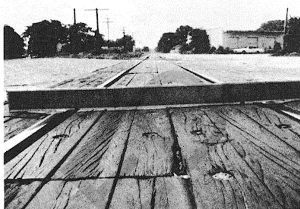
Figure B-53. Low-severity railroad crossing.
