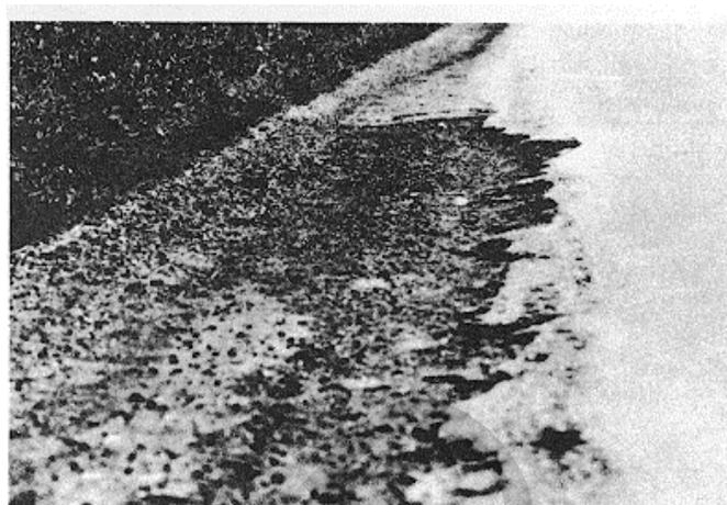
Figure B-30. High-severity edge cracking.
