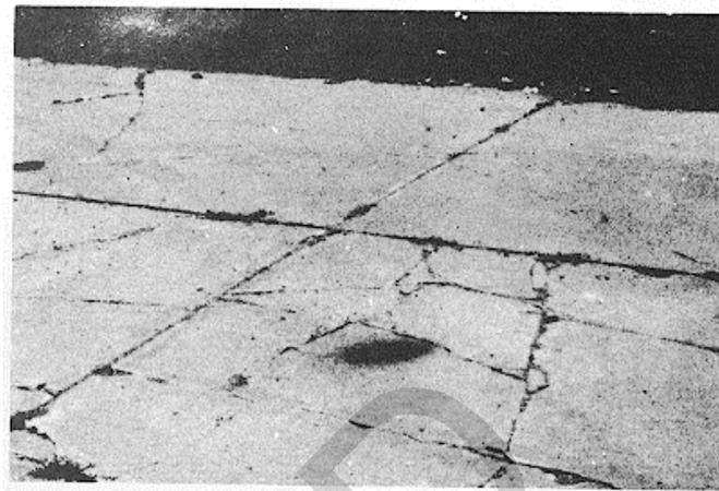
Figure B-82. High-severity divided slab caused by high-severity cracks.
