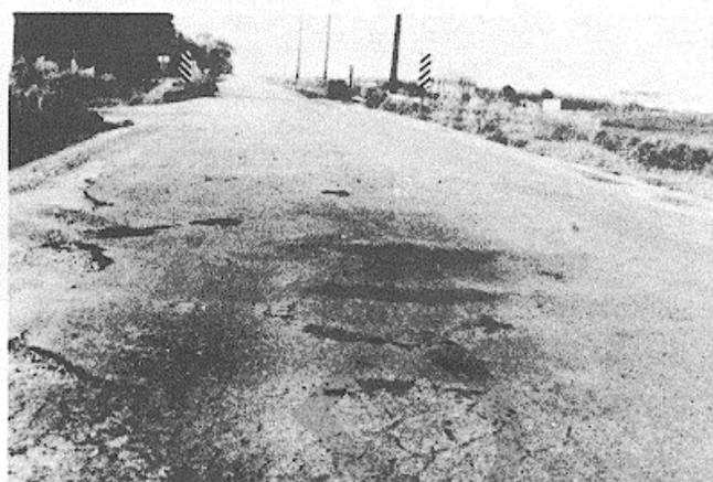
Figure B-61. Medium-severity shoving approaching high severity.
