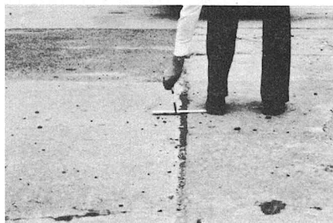
Figure B-91. Medium-severity faulting.
