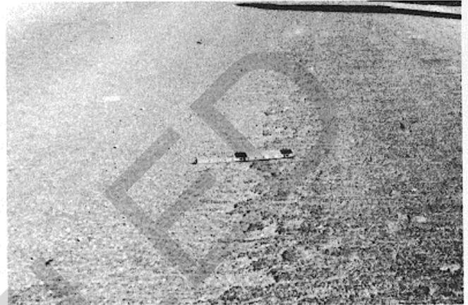
Figure B-68. Low-severity weathering and raveling caused by tracked vehicles.
