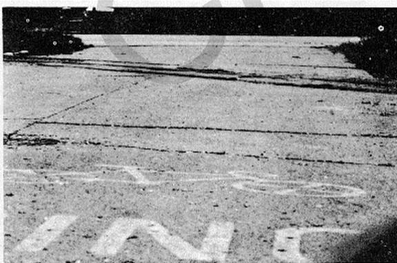
Figure B-124. Medium-severity railroad crossings.
