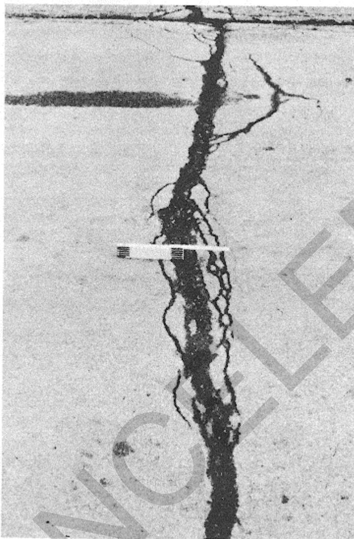
Figure B-33. High-severity joint reflection cracking.
