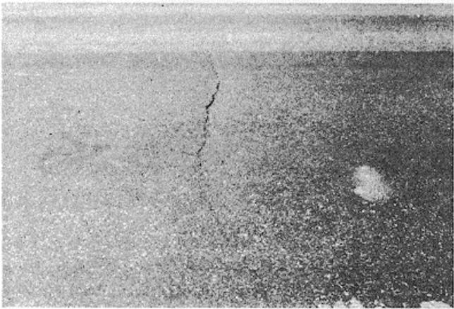
Figure B-38. Low-severity longitudinal and transverse cracking.
