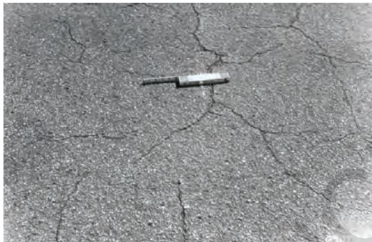
Figure 5.3. Low-severity block cracking
