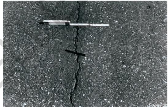
Figure 10.4. Medium-severity, longitudinal construction joint crack
