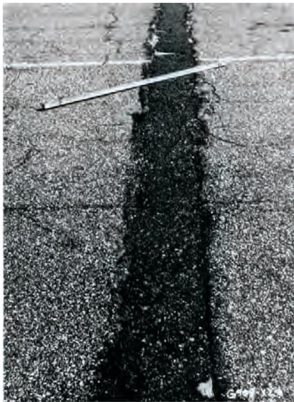
Figure 12.5. High-severity patch
