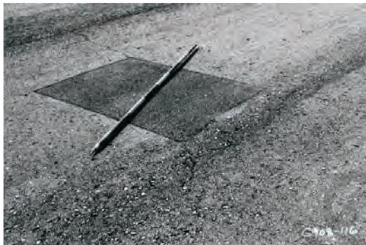
Figure 12.3. Low-severity patch
