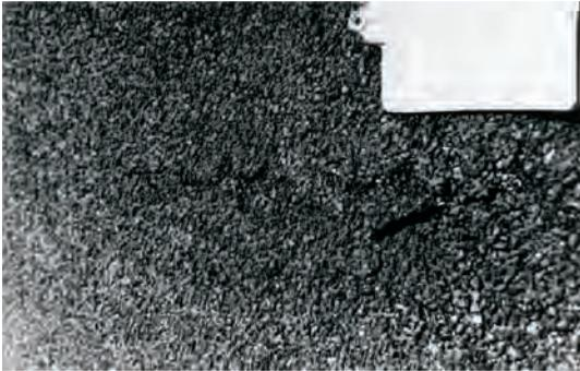
Figure 10.9. High-severity crack, PFC pavement
