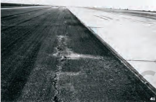
Figure 16.3. High-severity shoving
