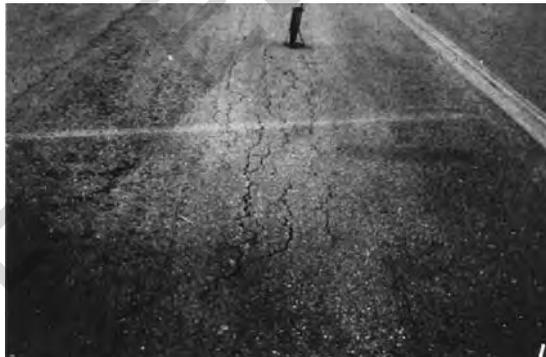
Figure 3.4. Low-severity alligator cracking, approaching medium severity
