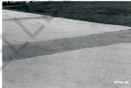
Figure 12.4. Medium-severity patch
