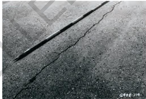
Figure 10.6. High-severity, longitudinal crack
