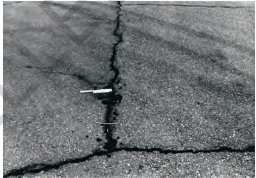
Figure 9.4. Medium-severity, joint-reflection cracking
