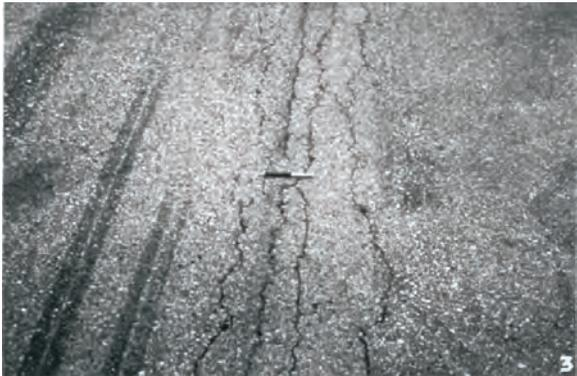
Figure 3.5. Medium-severity alligator cracking
