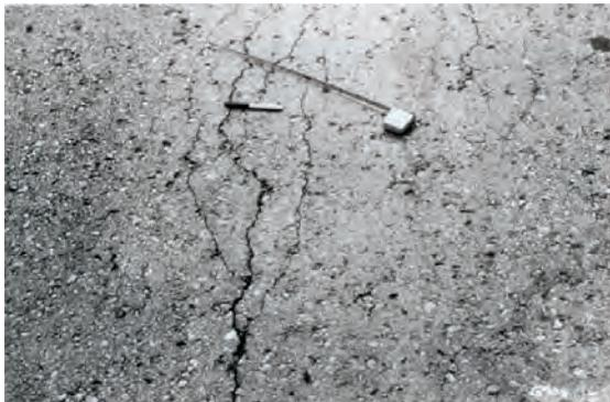
Figure 3.3. Low-severity alligator cracking
