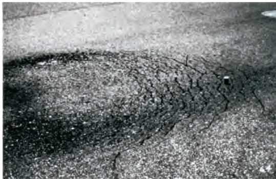
Figure 17.3. Slippage cracking
