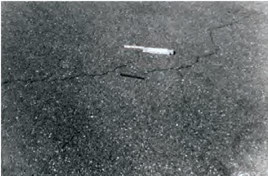
Figure 10.3. Low-severity, longitudinal cracks, approaching medium
