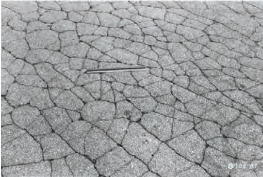
Figure 3.7. High-severity alligator cracking
