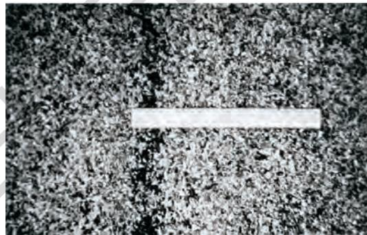
Figure 10.8. Medium-severity crack, PFC pavement
