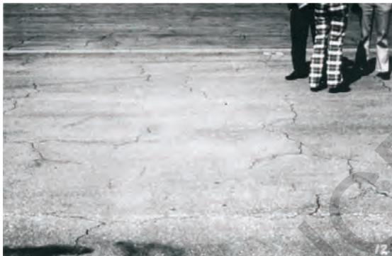
Figure 5.5. Medium-severity block cracking
