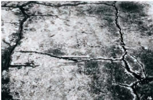
Figure 5.7. High-severity block cracking
