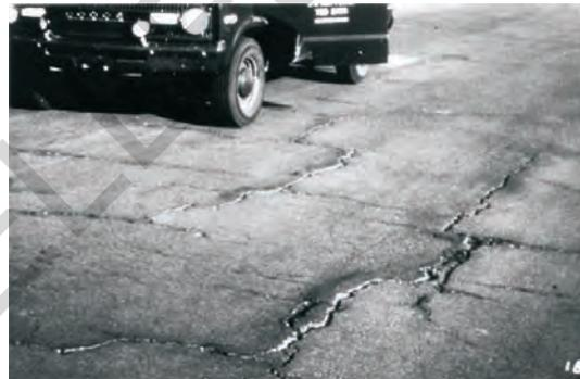
Figure 5.8. High-severity block cracking
