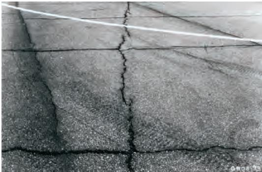
Figure 9.5. High-severity, joint-reflection cracking
