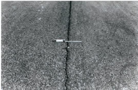
Figure 10.5. Medium-severity, longitudinal crack
