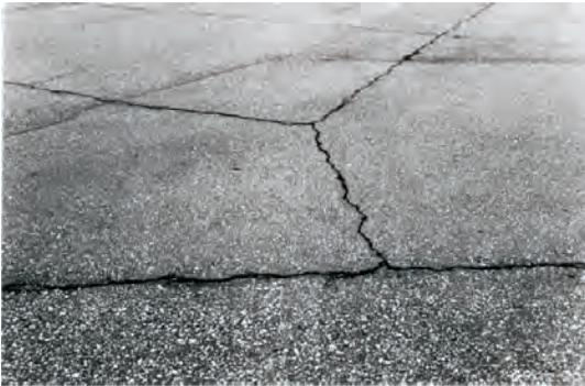
Figure 9.3. Medium-severity, joint-reflection cracking
