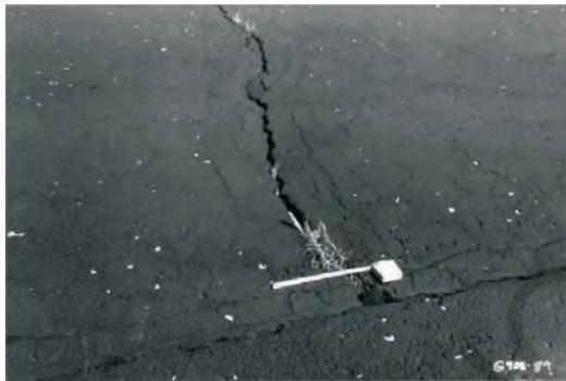
Figure 10.7. Low-severity crack, porous friction course (PFC) pavement
