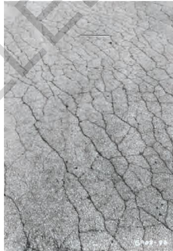
Figure 3.6. Medium-severity alligator cracking
