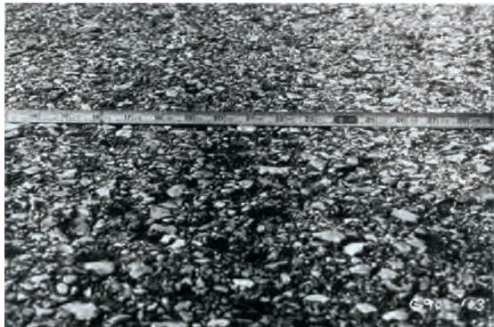
Figure 14.5. High-severity raveling/weathering
