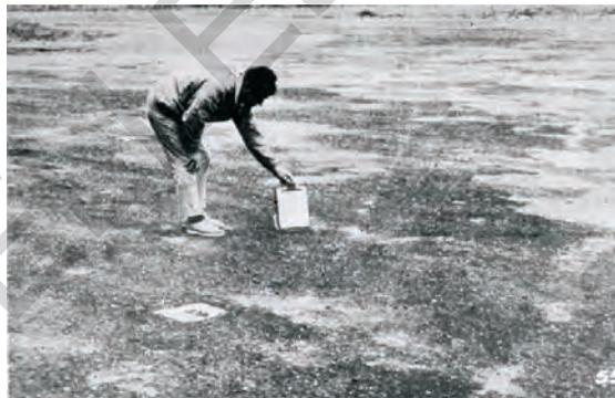
Figure 14.6. Typical PFC surface with no raveling and weathering
