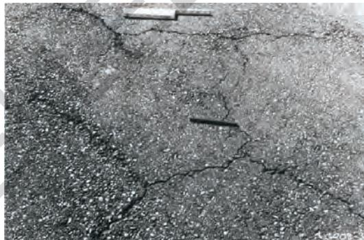
Figure 5.4. Low-severity block cracking
