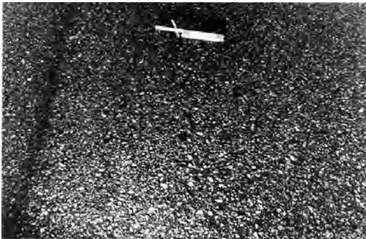
Figure 14.3. Low-severity raveling/weathering
