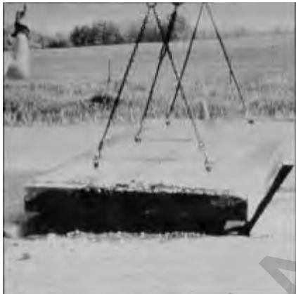
Figure 4.10. Pressure relief cut (lift-out method)
