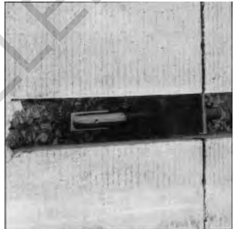
Figure 10.3. Core hole centered over crack
