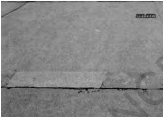
Figure 5.2. Severe spalling
