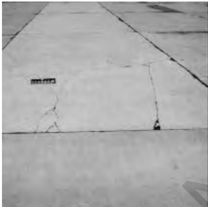
Figure 4.2. Bottom of deteriorated slab
