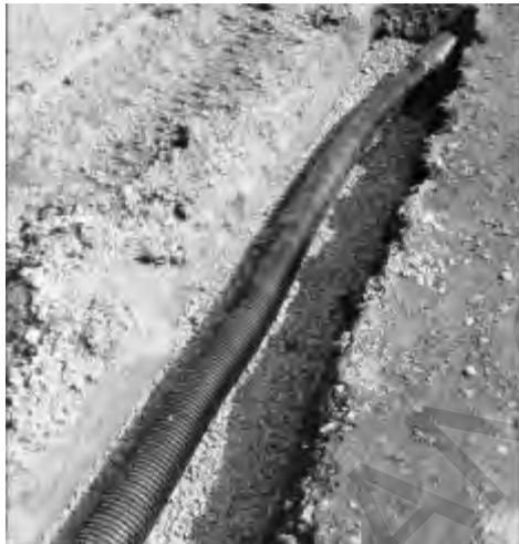
Figure 12.4. Filter fabric used to wrap collector pipe
