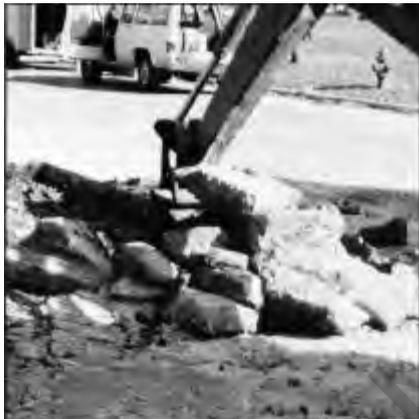
Figure 4.8. Additional saw cuts (breakup method)
