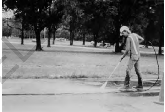
Figure 9.4. High-pressure water cleaning
