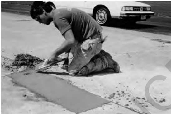
Figure 16.3. Finishing the patch surface
