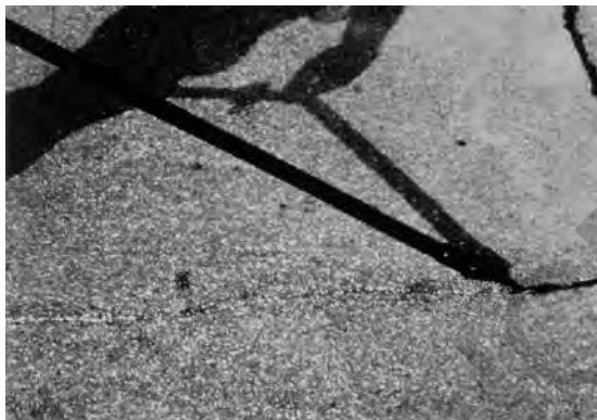
Figure 11.1. Sealing a crack
