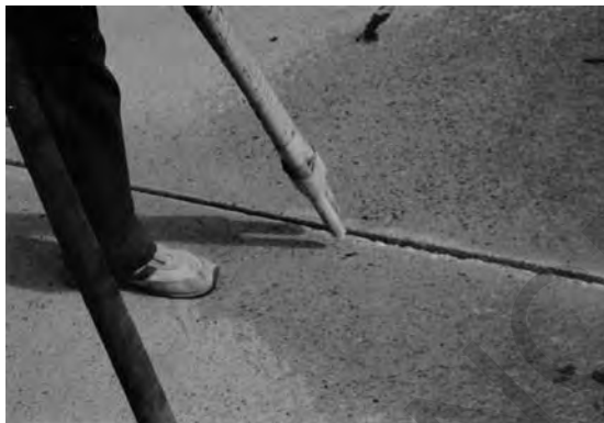
Figure 10.3. Sandblasting a joint face
