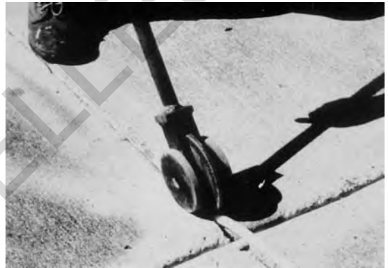
Figure 9.6. Installation of backer rod
