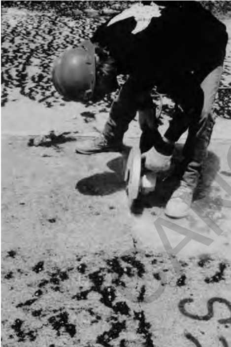
Figure 10.1. Hand sawing a crack
