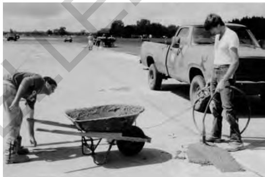
Figure 16.2. Consolidation of the repair material by vibration
