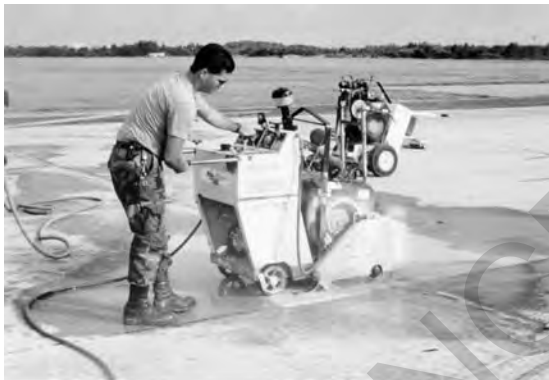
Figure 14.1. Sawing out the edges of a spalled area
