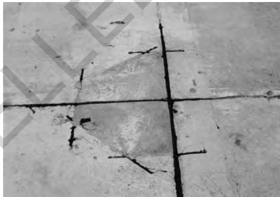
Figure 16.4. A completed spall repair that bridges an expansion joint
