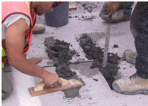
After consolidation and finishing, place a curing compound on the patching material to minimize rapid patch material shrinkage. Depending upon the type of repair material, the pavement may be opened to traffic in as little as a few hours. The minimum compressive strength required to open a repair to traffic is about 2,000 psi (13.7 megapascals) for slabs 8 inches (200 millimeters) or thicker.
