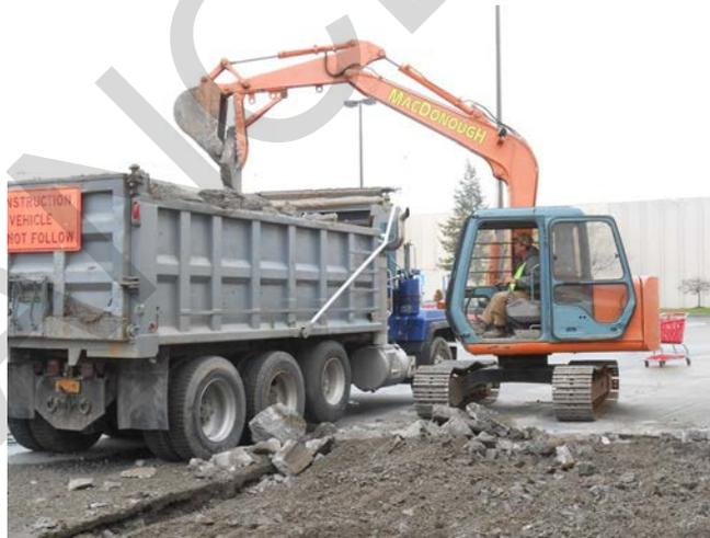
Figure 14-6 Additional Saw Cuts (Breakup Method)
