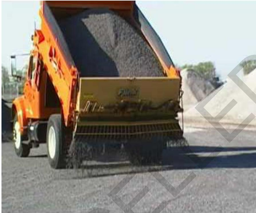
**Figure 6-2 Applying Aggregate with Self-Propelled Hopper-type Spreader**
