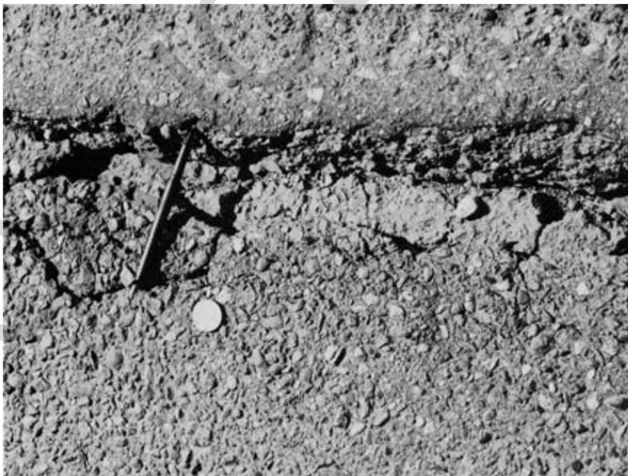
**Figure 9-8 Crack After Cleaning**
