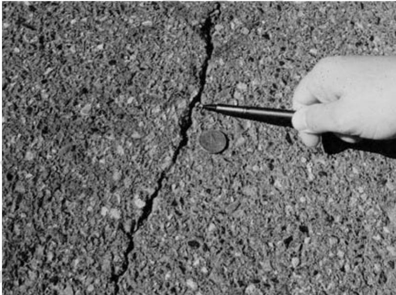
Figure 9-6 Medium Crack
