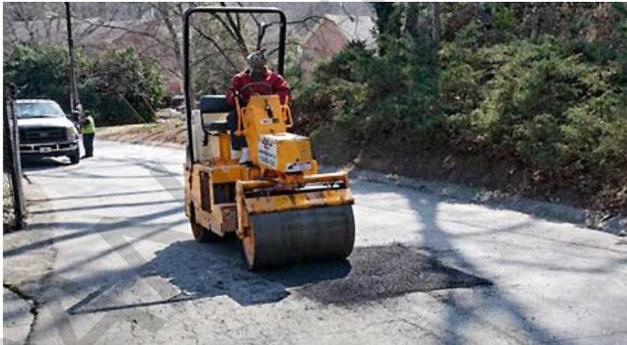
Figure 3-9 Check Level of Patch Surface
