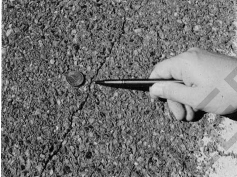
**Figure 9-5 Small Crack**
