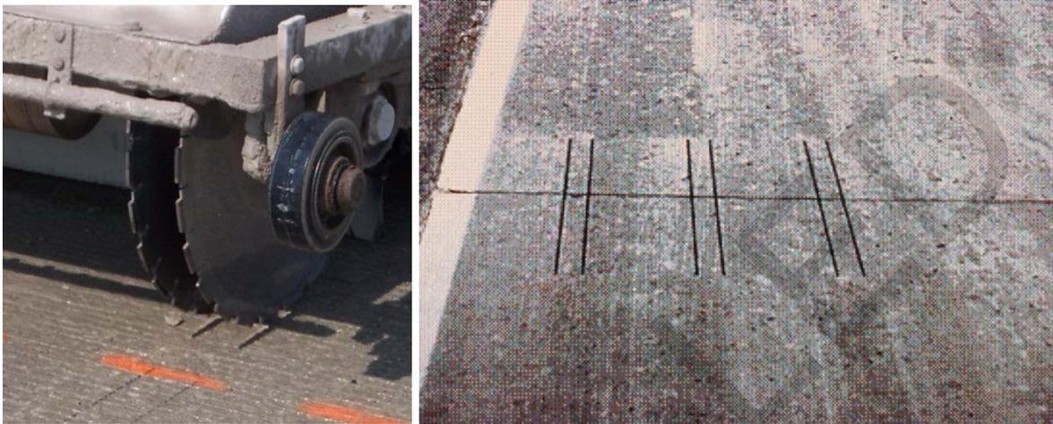
Where slab movement at the crack/joint location is required, cut slots to allow dowel placement parallel to the pavement surface at mid-depth and perpendicular to the orientation of the crack/joint.
