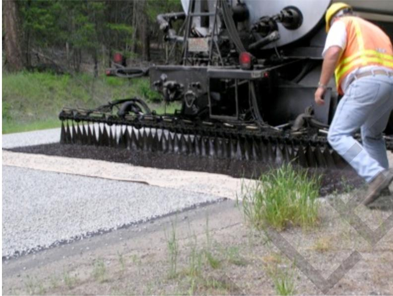
Figure 6-4 Aggregate and Sprayed Asphalt Spread Pattern
