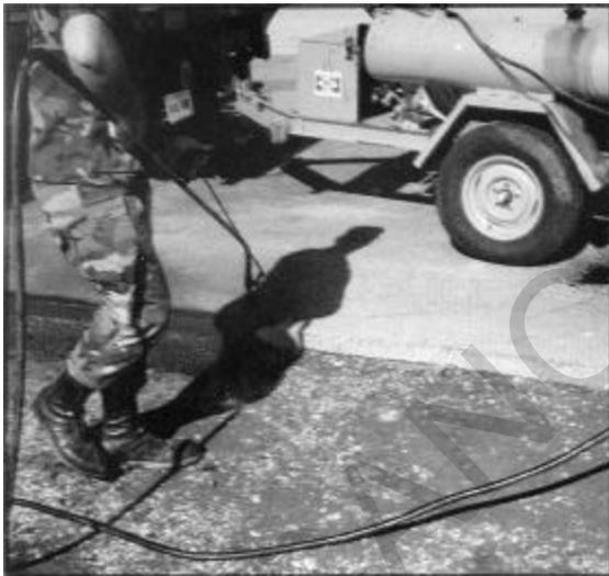
Figure 3.8. Overfilled patch area
