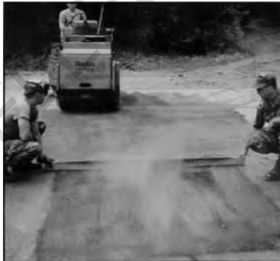
Figure 3.13. Sealing edges of the patch
