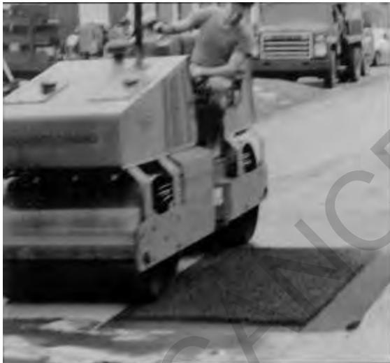
Figure 3.12. Level patch surface
