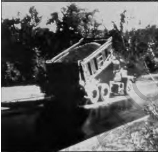
Figure 5.2. Applying aggregate with self-propelled hopper-type spreader
