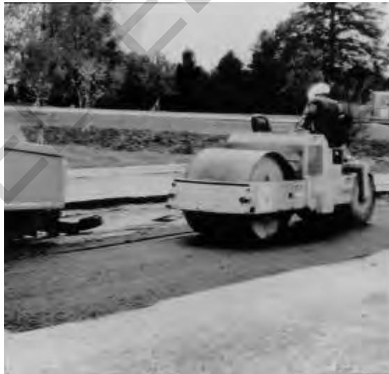
Figure 3.11. Overlapping compaction lanes
