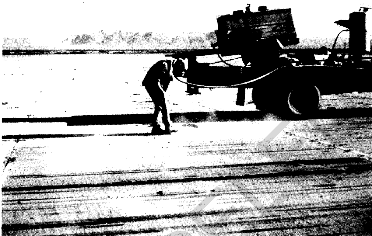
Figure 4-4. Sandblasting Equipment Cleaning Joints.
