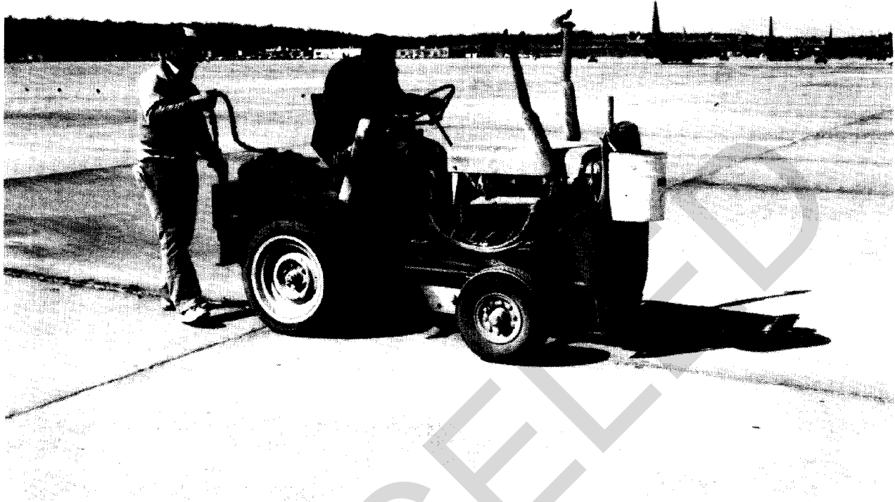
Figure 4-3. Joint Plow Removing Old Sealant.
