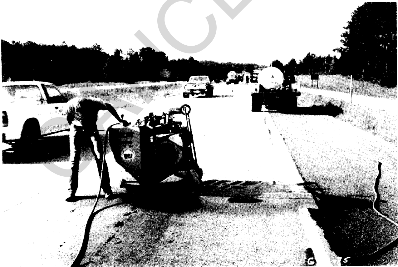
Figure 4-1. Concrete Saw Refacing Joint.
