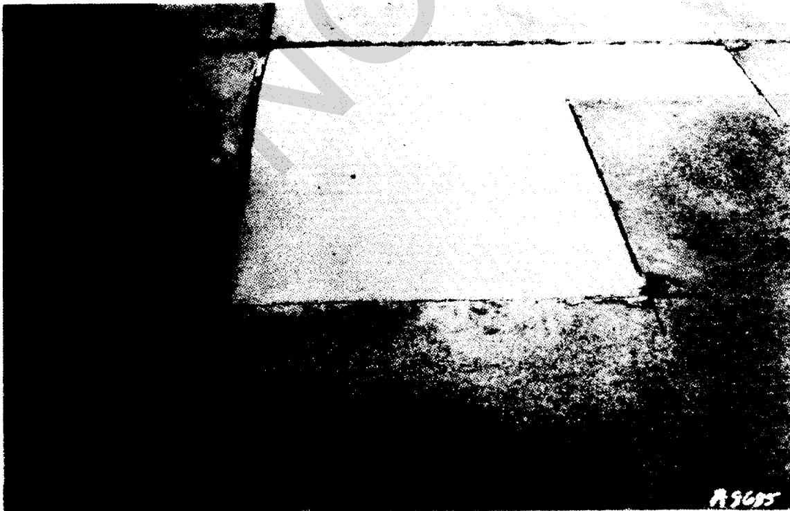
Figure 4-16. Example of a Rebuilt Joint.
