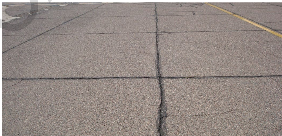
Figure 3-3 Reflective Cracking
