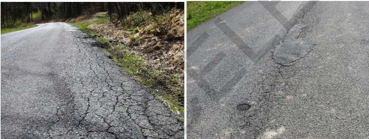
Figure 4-11 Good Pavement Candidates for FDR*
