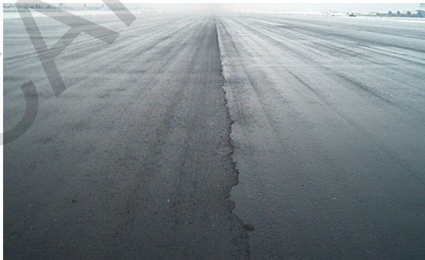
Figure 3-4 Longitudinal Cracking
