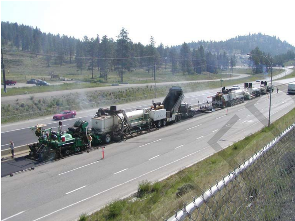
Figure 5-11 Example of Single Stage Remixing Train
