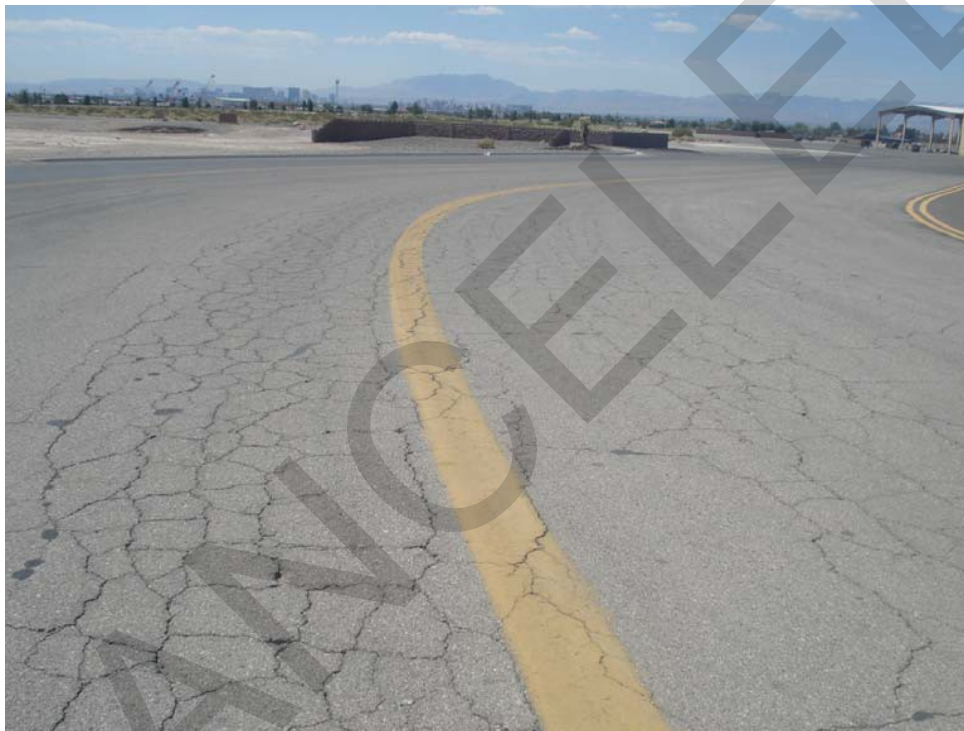
Figure 3-1 Alligator Cracking
