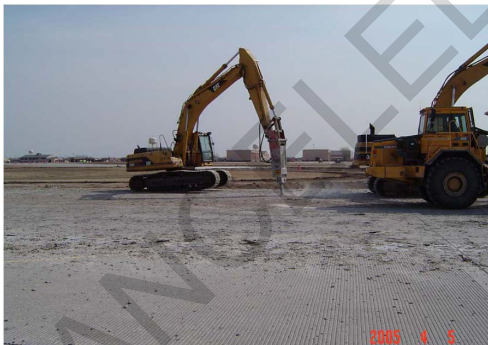
Figure 6-10 Excavator W/Hydraulic Impact Hammer (Ram Hoe) Attachment*
