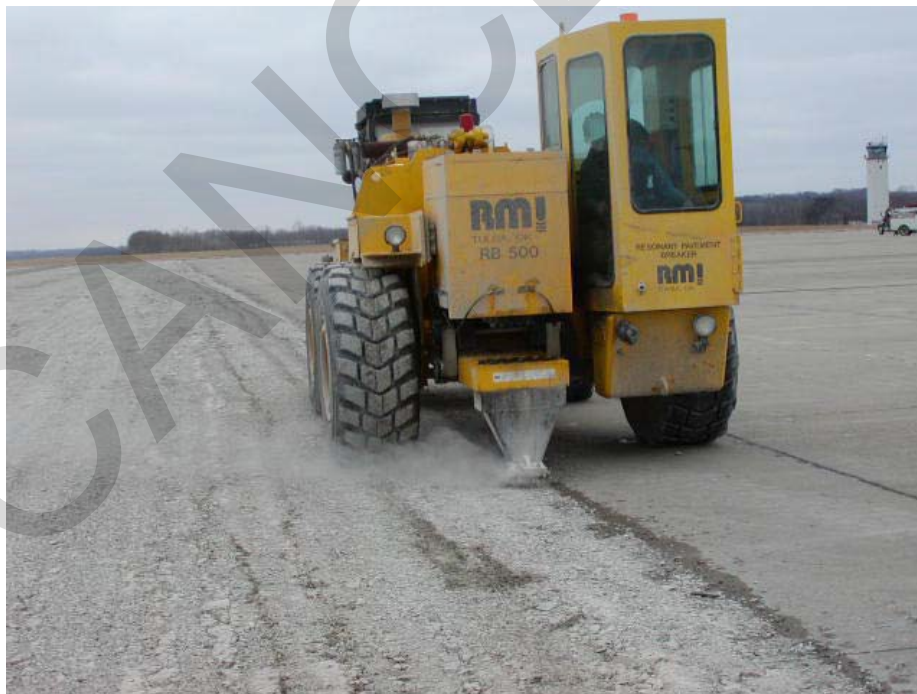
Figure 6-6 Rubblization Using RPB*
