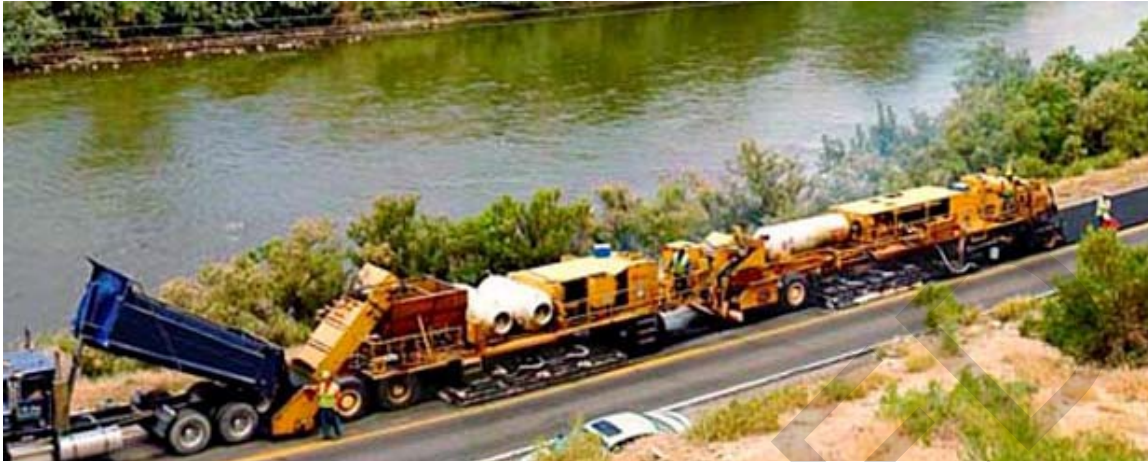
Figure 5-9 Surface Recycle Mix Placement*
