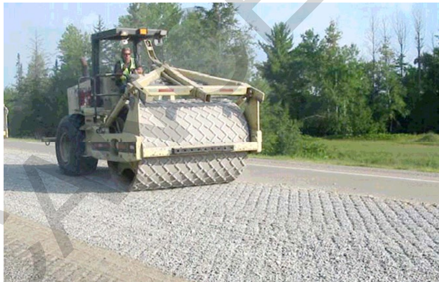
Figure 6-9 Z-Grid Roller Used on MHB Rubblized Pavement*
