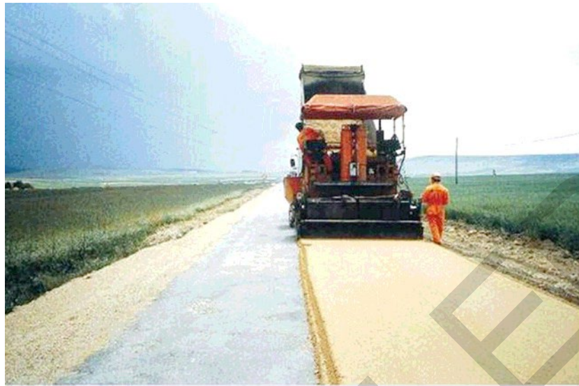
Figure 4-12 Granular Material Added to Achieve Compacted Thickness*
