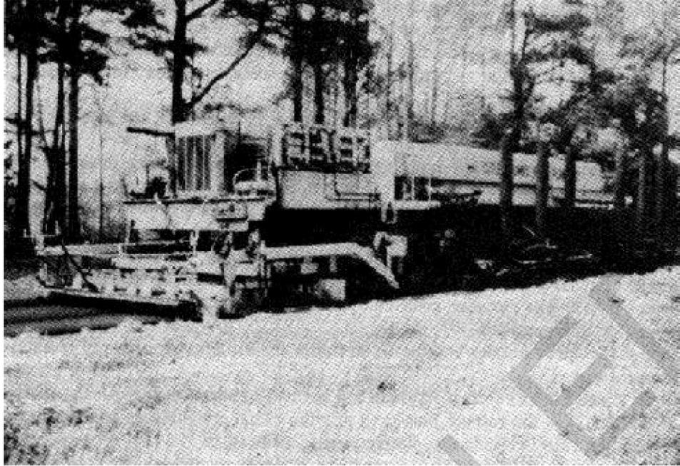
Figure 2-3. Self-contained heater-planer.
