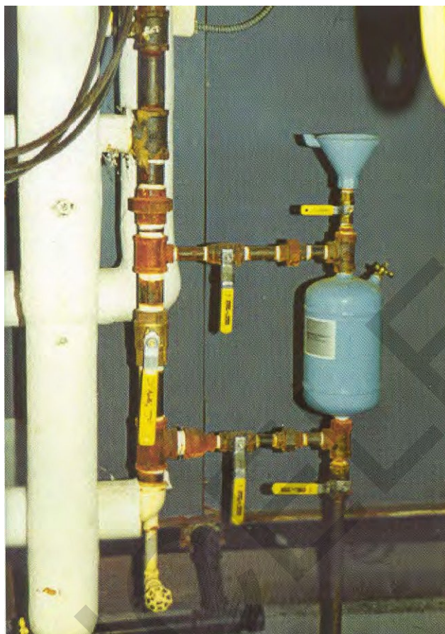
Figure 8-1 Chemical Pot Feeder
