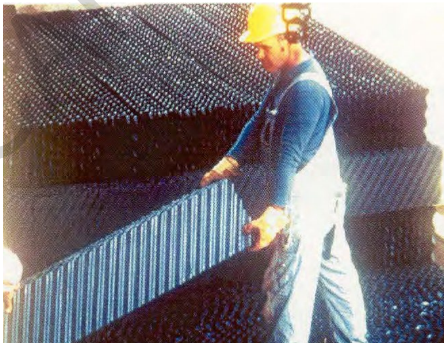
Figure 5-11 High-Efficiency Cooling Tower Film Fill
