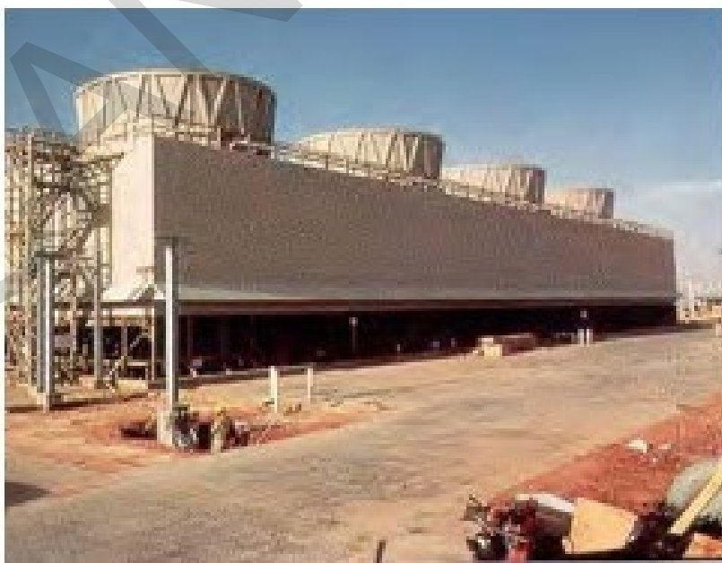
Figure 5-9 Counter-Flow Cooling Tower
