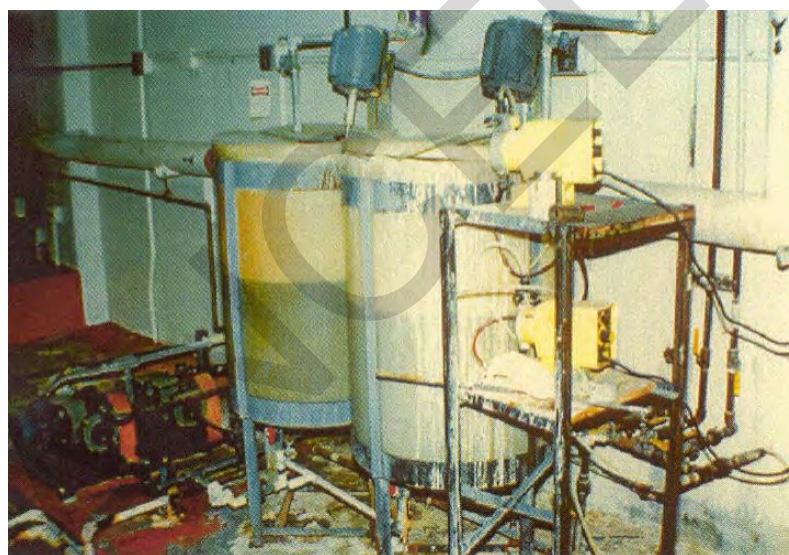
Figure 8-3 Automatic Chemical Feed System
