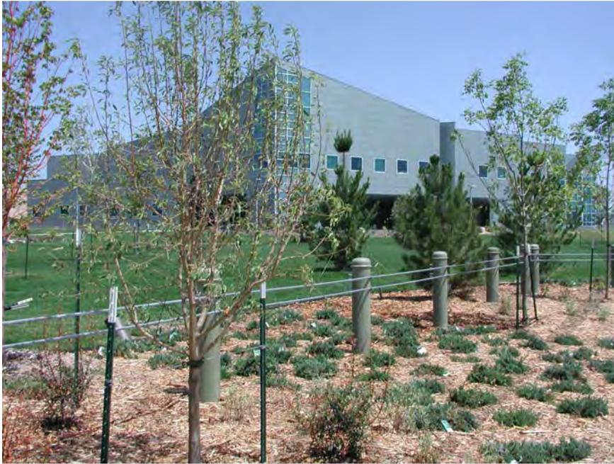
If site furnishings are hardened to provide crash resistance and are placed with approved spacing, they can be incorporated as part of the perimeter design. \1\UFC 4-010-01/1/ provides guidance on the types of site furnishings that are prohibited and what types are allowed if properly hardened. Specific types of site furnishings to consider for the purpose of security design are:
