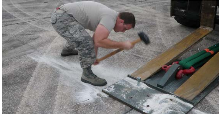
Figure 3-14. Drill Holes and Install Anchors at Back of Plate.
