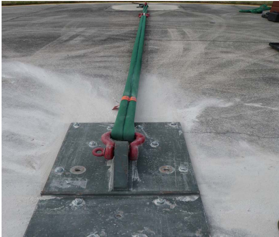
Figure 3-16. Complete Installation of Anchors.
