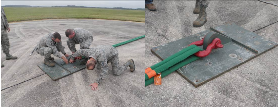
Figure 3-10. Connect Sling to Steel Plate.
