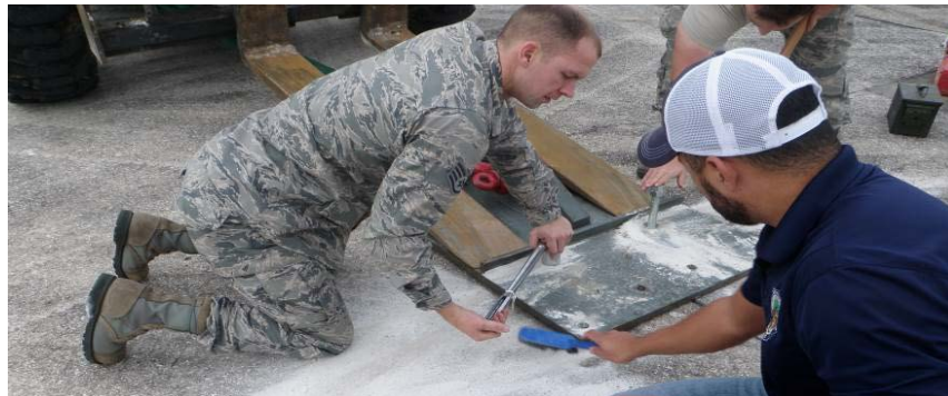
Figure 3-15. Install Seven Anchors at Back of Plate.
