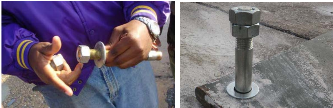
Figure 3-12. Assemble Anchor Bolts.
