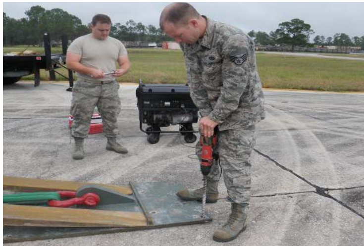
Figure 3-13. Use Forklift to Hold Plate while Anchoring.
