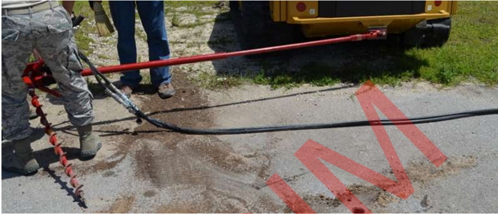
Figure 3.8. Torque Converter Connection.
