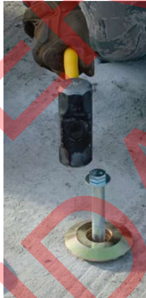
Figure 3.15. Heavy Duty Sleeve Anchor Placement.
