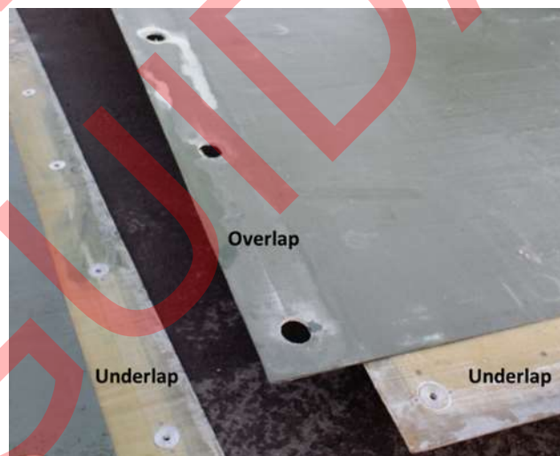
Figure 2.4. FRP Panel Overlap/Underlap Edges.
