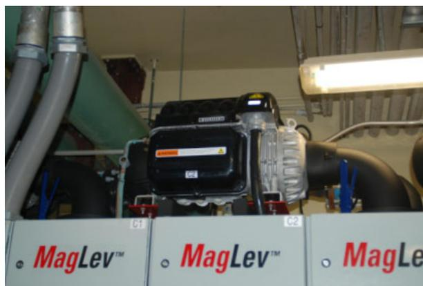
*Turbocor pumps provide an oil-less solution in mitigating corrosion (Navy Hospital Guam).*
