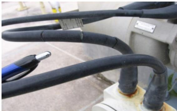
*According to the definition outlined by Congress, ultraviolet (UV) deterioration of electrical wire insulation is considered corrosion.*
