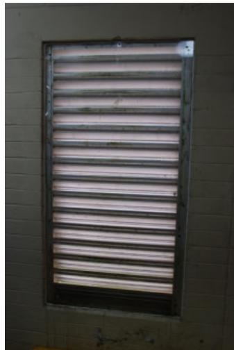
*Local standards in Guam call for sealing intake of chiller rooms to mitigate corrosion.*
