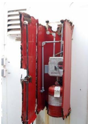
*This corroded fire extinguishing system could be elevated as a safety priority.*
