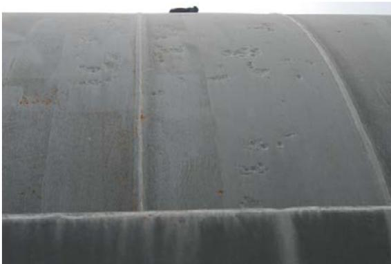
*Pitting corrosion on a fuel tank, Guam.*
