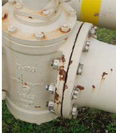
*SRM fuels pipeline requires recoating to prevent further corrosion.*
