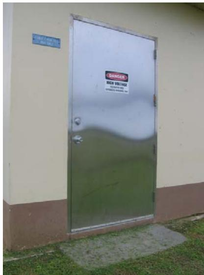
*An example of a corrosion-resistant stainless steel door in a high ESI zone (Guam).*
