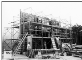
Built-in-place formwork
