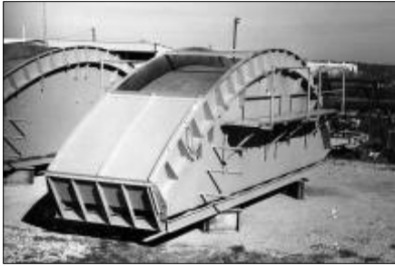
TechSpan Arch forms are fixed to the dimensions of the magazine
