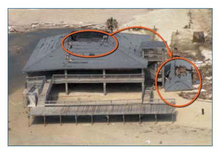
FIGURE 2-2: Roof structure failure on a house (Galveston, TX, 2008) (SOURCE: FEMA P-757) buildings suffered wind damage, some of which was disproportionate to the reported wind speeds. During Hurricane Ike, the house in Figure 2-2 sustained structural damage from wind speeds estimated at 93 mph, which was below the design wind speed.
