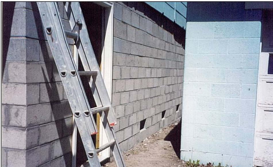
**Figure 8-3. New foundation with vents**
