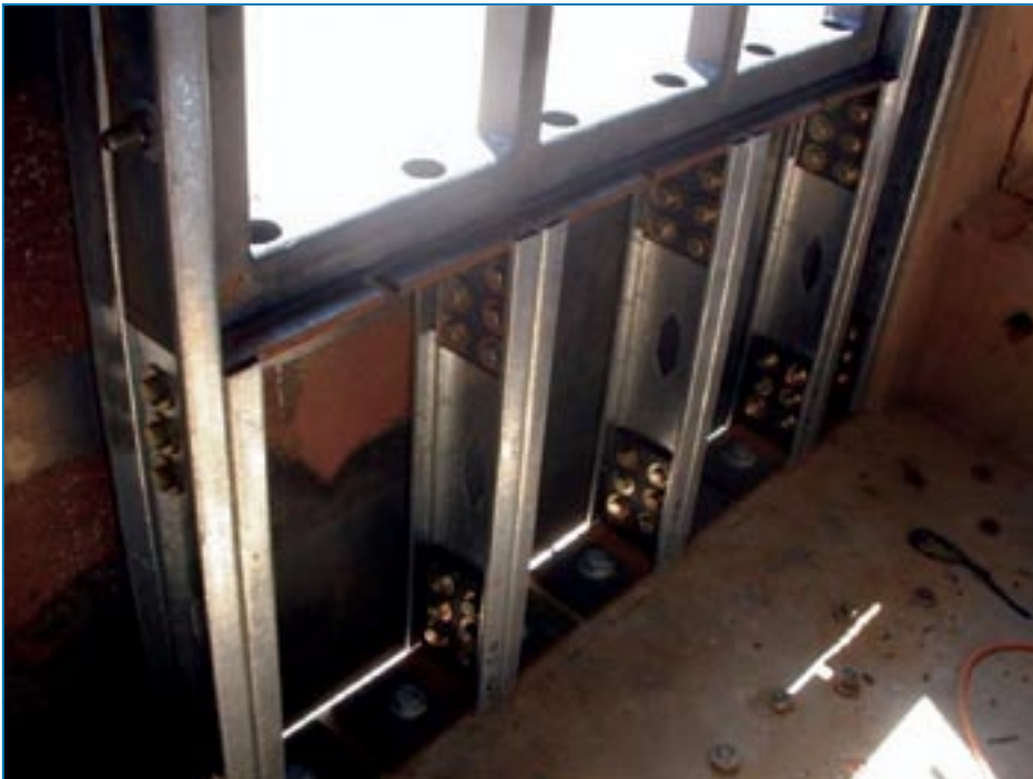
Figure 3-12: Metal stud blast wall.
