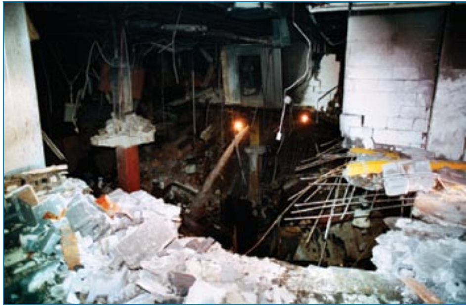
Figure 3-1: Damage in WTC garage caused by the 1993 bomb attack.
