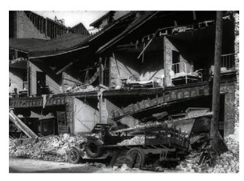
Figure 6-2: Santa Barbara, 1925, typical failure of brick walls and timber interior.
