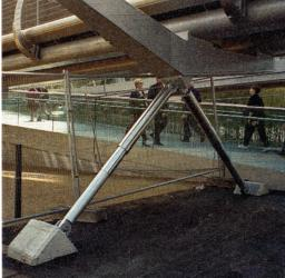
Figure 5-44: Elegantly expressed exposed bracing: Left: University Administration Building, Berkeley California, Architect: Hansen Murakami and Eshima. Right: Millenium Bridge, London, 2000. Architect: Foster Associates; Arup Engineers, Engineer.
