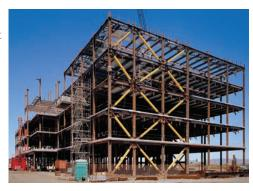
4. Coupled 3-part systems with moment frames, links, and shear walls to provide a progressive resistance system in which the resistance progresses from the most rigid system to the more ductile-flexible system.
