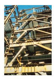
2. The dual-system steel-moment frame and passive seismic dampers provide high damping, which significantly reduces the seismic loads imparted to the moment frame.
