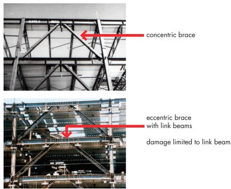
with interior eccentric-braced frames. Another variation is the use of shear walls combined with a moment-resistant frame in which the frames are designed to act as a fail-safe back-up in case of shear-wall failure.
