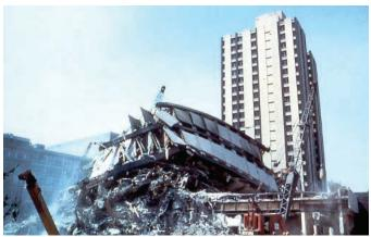
suffered moderate damage. The structures had asymmetrical lateral bracing at their perimeters, and the steel frames were poorly detailed and buckled (Figure 5-26).
