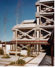
Figure 5-42: Exposed cross-bracing examples.
