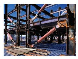
3. **Unbonded steel braces** with the brace providing stable tension-compression behavior, a significant improvement over the conventional braced frame.
