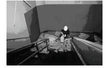
Figure 9-6: Difficulty in exiting due to debris strewn across exit stairs can be an indirect threat to life, as can be seen in this photo following the Loma Prieta earthquake in 1989.
