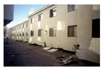
Figure 8-5: A tuck-under similar to Figure 8-4, but much more modern and designed at a time when the weakness of the parking level was more understood. In this case, the detailing of the small wood shear walls at that level was poor. This practice created another set of deficient "existing" buildings.
