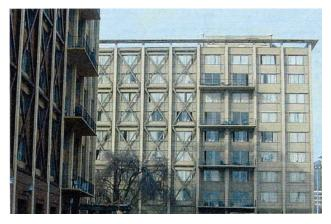
Figure 5-43: Left: Retrofitted student residences. Right: University Administration Building, Berkeley California, Architect: Hansen, Murakami and Eshima, Engineers; Degenkolb Engineers.
