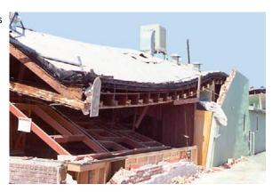
characteristics that lead to poor performance were allowed over the years. For example, concrete buildings of all types were economical and popular on the West Coast in the 1950s and 1960s. Unfortunately, seismic provisions for these buildings were inadequate at the time, and many of these buildings require retrofit. Highlights of inadequacies in past building codes that have, in many cases, created poor buildings are given below.
