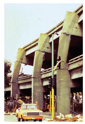
Figure 6-6: San Francisco, 1989, elevated highway support bents, an example of failure of engineered structures.
