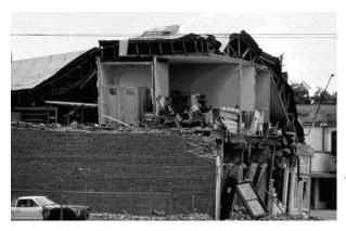
Figure 9-4: Nonstructural partition walls prevented the total collapse of this unreinforced masonry structure in the 1983 Coalinga earthquake.
