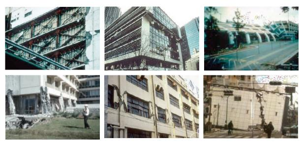
Figure 7-12: Examples of typical earthquake damage.
