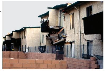
Figure 5-10 shows another apartment house in Northridge in which two stories of wood frame construction were supported on a precast concrete frame. The frame collapsed completely. Fortunately there were no ground floor apartments, so the residents, though severely shaken, were uninjured.
