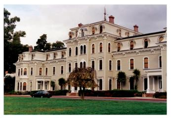
Figure 8-21: Mills Hall, Mills College, California. Structure is wood studs and sheathing. Interior shear walls were created by installing plywood on selected interior surfaces.
