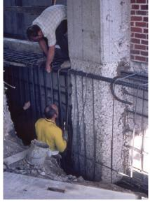
Figure 8-11: Retrofit activities inside buildings are most often not surgical or delicate. Here work on a new foundation for a shear wall is prepared for casting.
