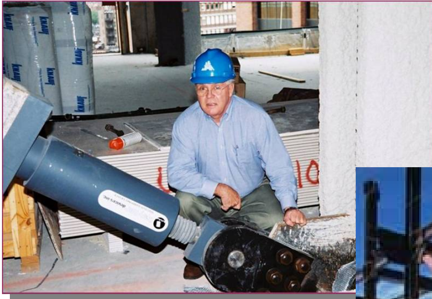
Huntington Tower Boston, MA
