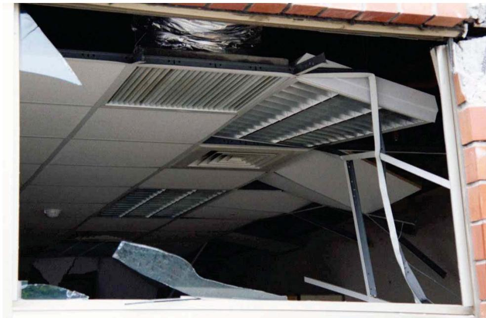
Figure C13.1-4 Damaged ceiling system.
