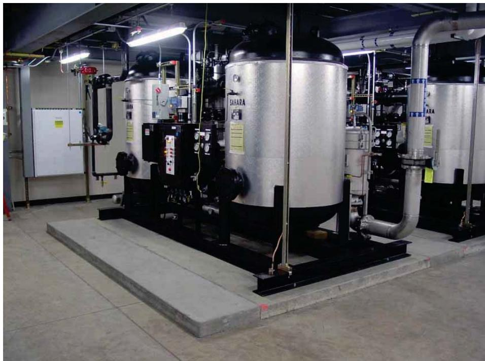
Figure C13.1-6 Skid-mounted components.
