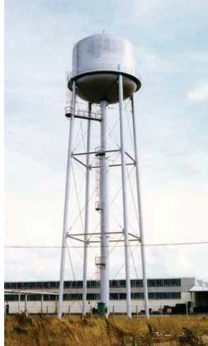
Figure C15.7-1 Multi-leg braced steel tank.
