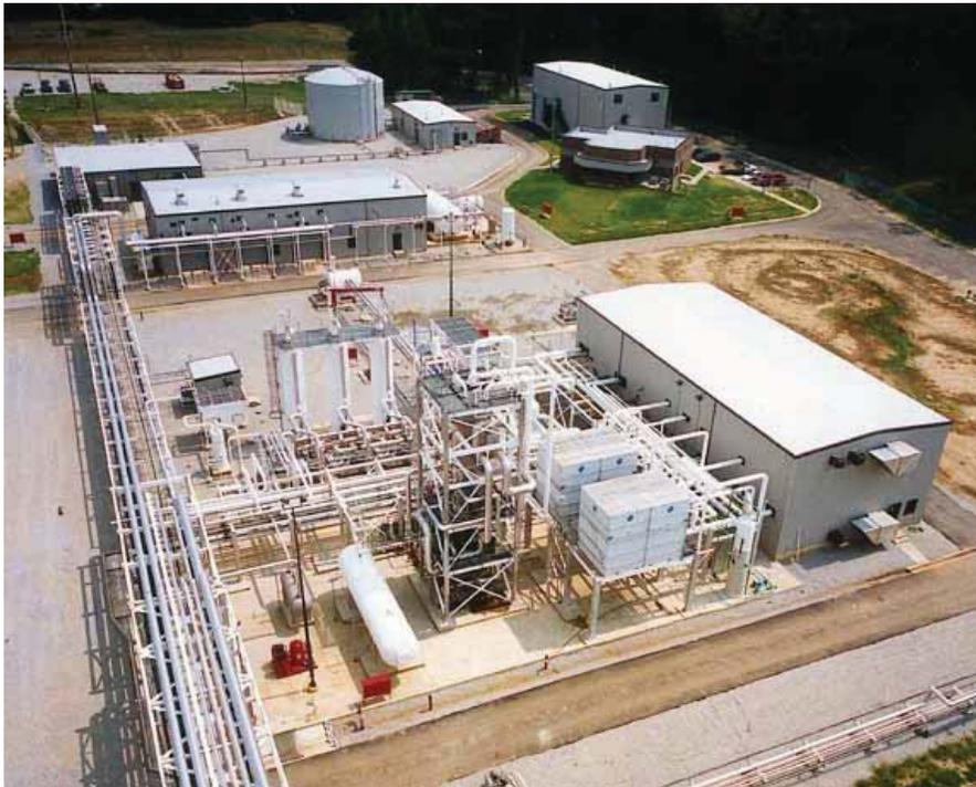
Figure C15.1-2 Steel pipe rack.
