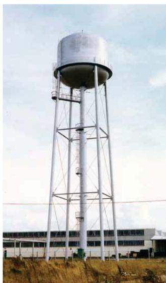
Figure C15.1-1 Steel multi-legged water tower.
