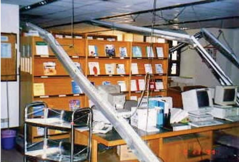
Figure C13.1-2 Collapsed light fixtures.
