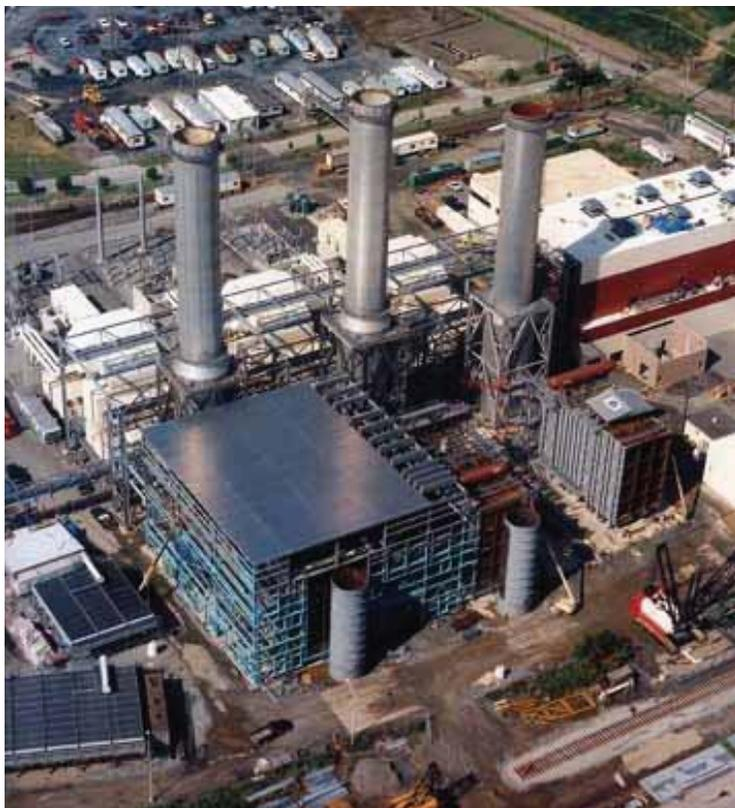
Figure C15.1-3 Heat recovery steam generators.
