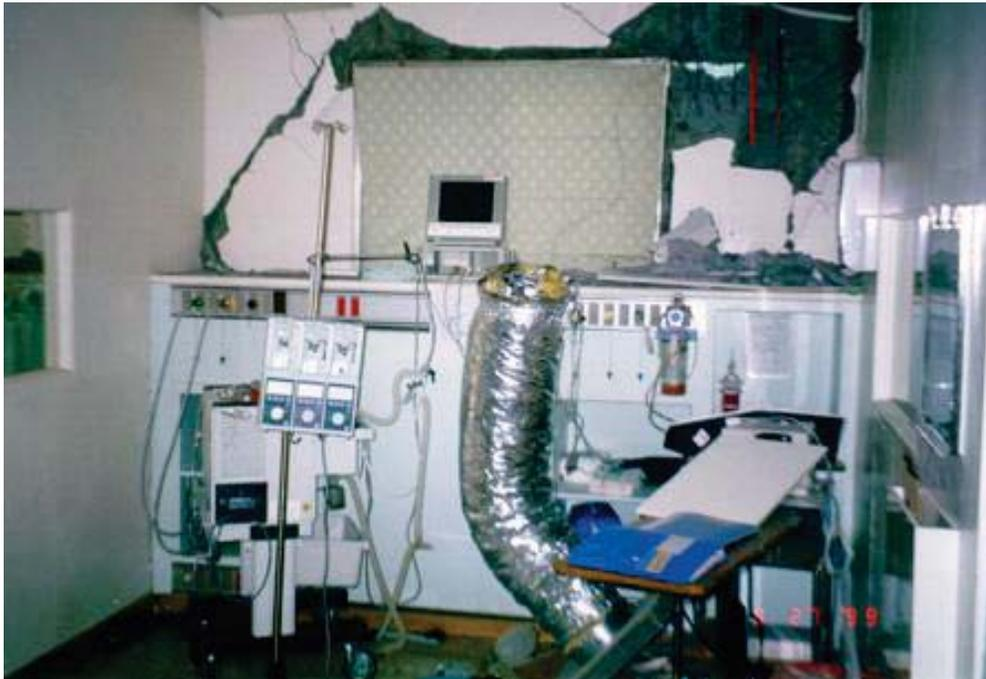
Figure C13.1-3 Collapsed duct and HVAC diffuser.
