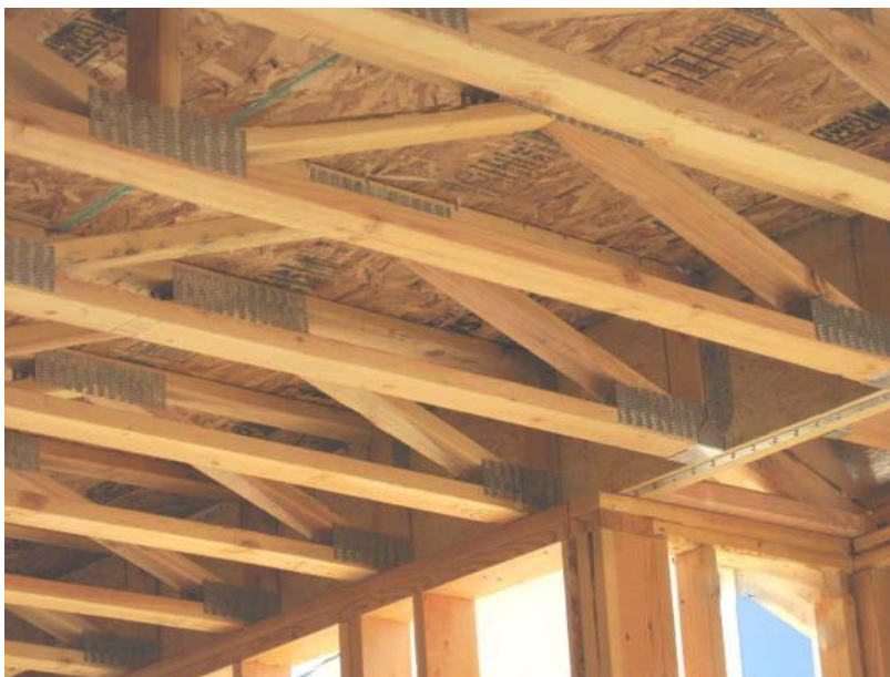
FIGURE 6-6 OSB floor diaphragm on engineered wood trusses
