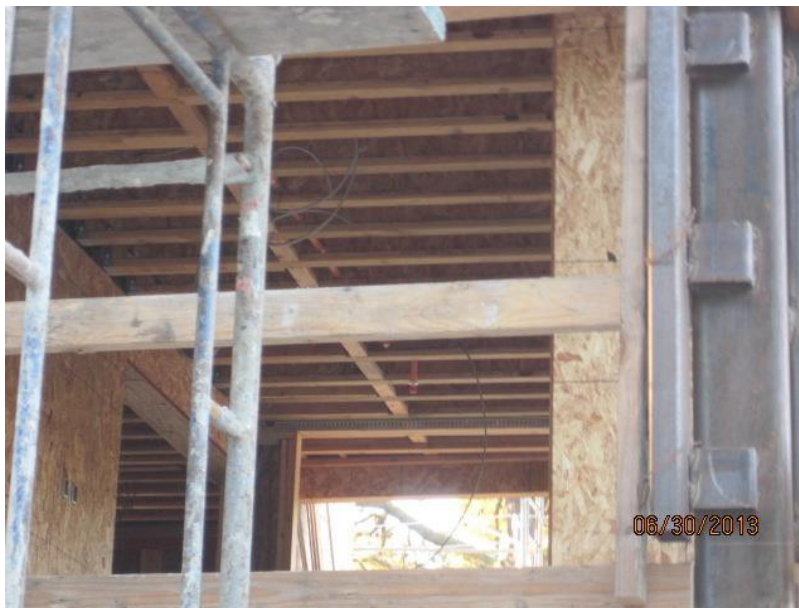
FIGURE 6-5 I-joist framing members
