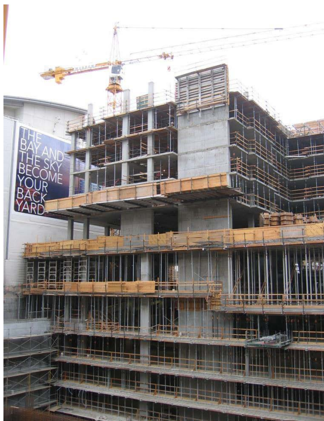
FIGURE 3-3 A shear wall in a concrete structure
