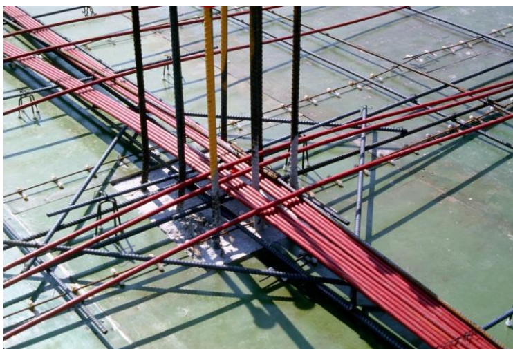
FIGURE 3-2 Post-Tensioned Slab Reinforcement at Column
