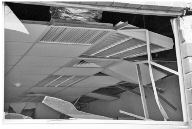
FIGURE C13.1-4 Damaged Ceiling System
