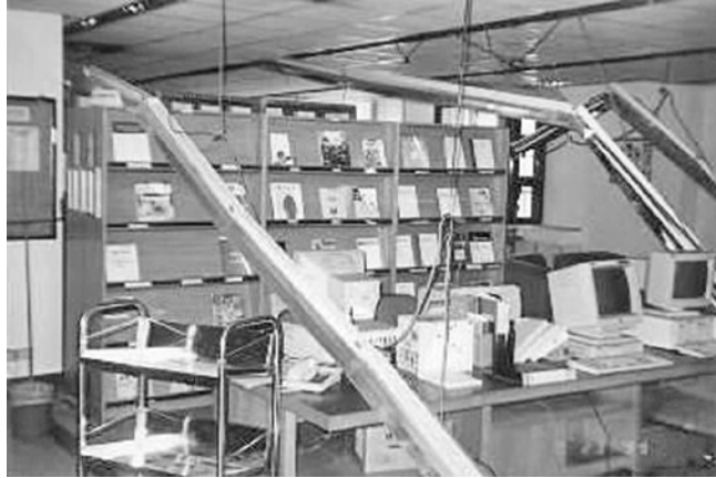
FIGURE C13.1-2 Collapsed Light Fixtures
