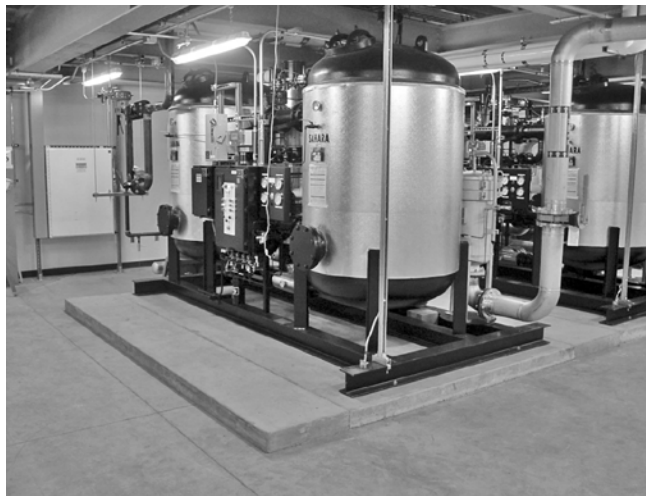
FIGURE C13.1-6 Skid-Mounted Components
