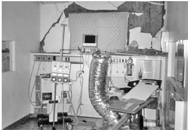
FIGURE C13.1-3 Collapsed Duct and HVAC Diffuser
