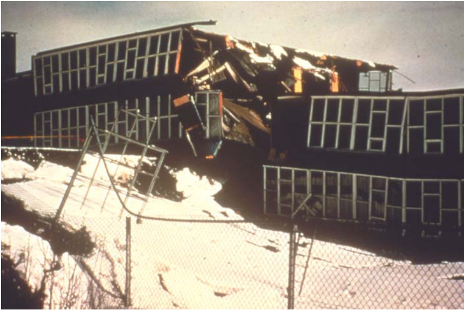
Figure 3-10 Government Hill School, Anchorage, destroyed by landslide during the magnitude-8.4 Alaska earthquake of 1964. (Photo courtesy of National Oceanic and Atmospheric Administration, National Data Service).
