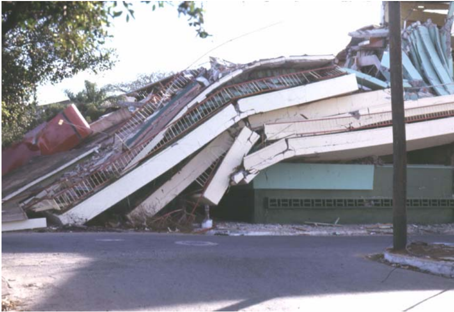
Figure 3-3 Older five-story reinforced concrete frame building in Managua, Nicaragua, that had inadequate seismic resistance and collapsed during the magnitude-6.2 earthquake of December 23, 1972. (photo courtesy of C. Rojahn)
