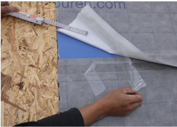
The boards come with an installed secondary water barrier. At the joints between the boards, the barriers are taped to each other (top over bottom barrier)
