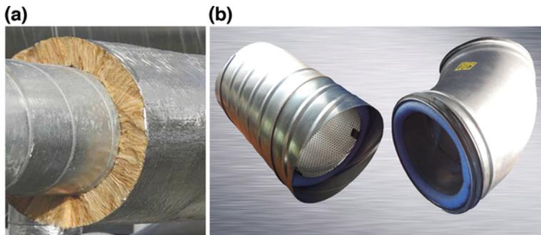
**Fig. 12.10** Examples of supply duct insulation: (a) external duct insulation (courtesy of Isover-Saint-Gobain), (b) internal duct insulation (courtesy of Linx Industries, Inc., Division of DMI)
