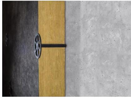
Fixation of insulation panels by special fastener
