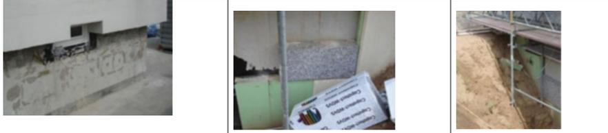
Basement walls are insulated over the water barrier using water-resistant XPS insulation boards. These boards are bonded jointless close to each other with a special waterproof adhesive. XPS boards are highly pressure resistant
