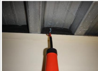
Testing roof/wall once section completed with air sealing foam tape
