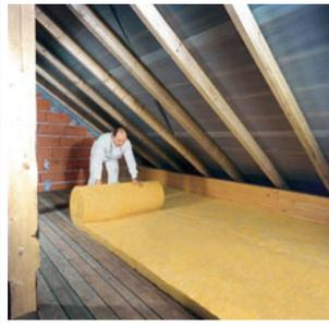
Batts and rolls are available in widths suited to standard spacing of wall studs, attic trusses or rafters, and floor joists. Note the batt insulation in between the roof rafters.
