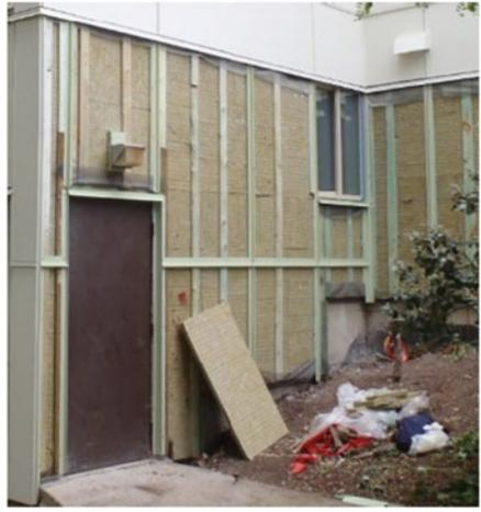
**Fig. C.10** Exterior insulation (EIFS) fastened with long screws through wood strapping (wood frame structure)
