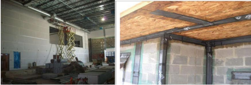
**Fig. 9.9** Gypsum air barrier partition wall used to compartmentalize an interior space: Left, see rear wall; Right, CMU and OSB sheathing is used as an air barrier assembly. (Photo courtesy of Nicholas Alexander, USACE)
