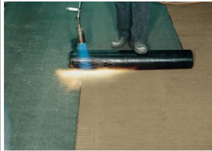
Flat roof insulation (stonewool) with direct glued bitumen sheeting
