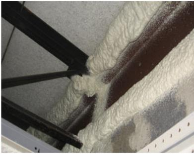
Roof/wall with cementitious wood fiber deck with purlins on CMU wall above ceiling tiles (foamed)
