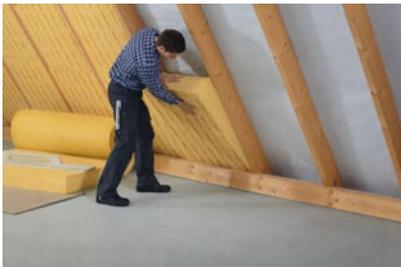
2. Install insulation panel between rafters; it clamps without additional fixation
