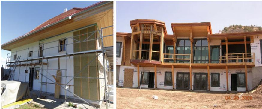
**Fig. C.16** Mechanically fixed to battens in strip or blanket format to increase R-value and reduce repeat thermal bridging through studs
