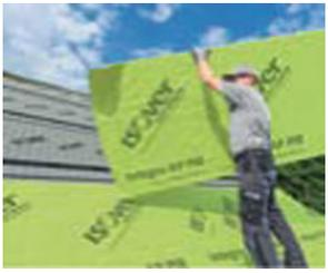
6a. Install the insulation layer of PIR, wood fiber, or mineral wool boards above the rafters
