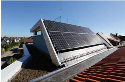
Finished roof with PV panels installed. The PV panels also act as mechanical fastening for the PUR boards and the rain barrier
