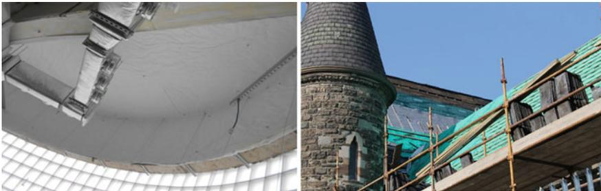
**Fig. C.21** Mechanically fixed to/through battens. Hygro-thermal risk assessment is recommended, particularly in heritage applications
