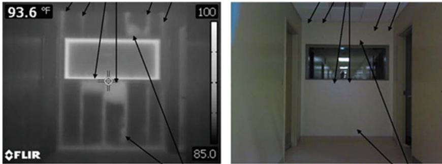
**Fig. H4.5** Loss of thermal barrier continuity through voids at missing insulation and thermal bridging through studs and air leakage under induced pressure differential. Note straight edge and irregular shape anomalies. Source: TMI Air Barrier Testing
