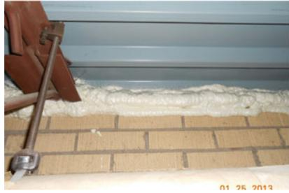
Roof/wall intersection air sealing completed with polyurethane foam
