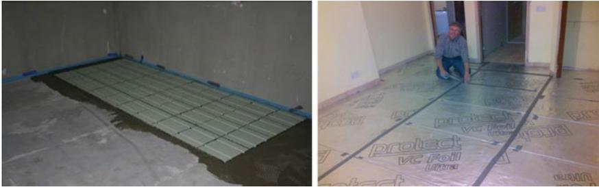
**Fig. C.20** Loose lay or panel application, suitable for domestic loadings. Address heat loss through concrete slab without requiring door/threshold adjustments
