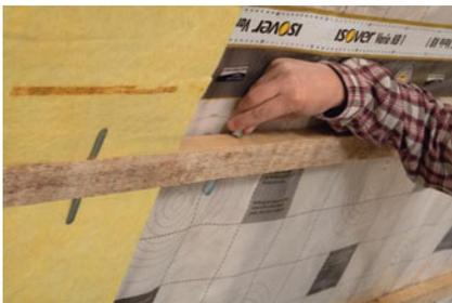
7. After installing and tightening the vapor barrier, attach it to the wooden studs to form a tight interior lining
