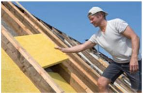
2b. Put a thin insulation layer on the existing inside lining. This protects the following vapor retarder from damaging by nails or screws
