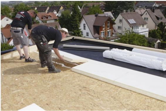
PUR rigid boards are placed upon the wooden roof construction and are secured in place (during the installation) by stripes of PUR spray foam. The boards are then covered by bitumen felt (and later with gravel, concrete pavement blocks or substrate for the roof garden)
