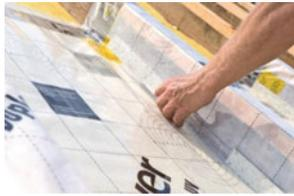
4b. Fix the vapor retarder close into the corner of the rafters by using small battens
