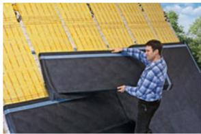
6b. Install the insulation layer of PIR, wood fiber, or mineral wool boards above the rafters
