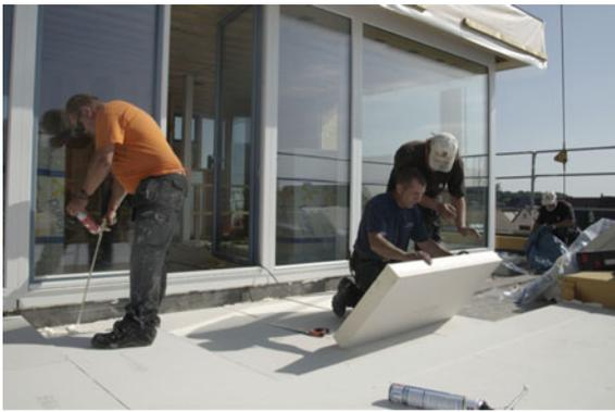
PUR rigid boards are placed upon the wooden roof construction in two layers and are secured in place (during the installation) by stripes of PUR spray foam
