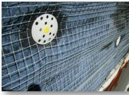
**Fig. C.15** Mechanical fixing (Polymer) of IWI thermal bridging assembly at window reveal (Aerogel Blanket, Vapor Barrier + MGO board)
