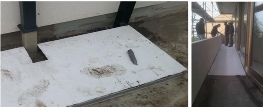
**Fig. C.19** Loose lay, adhesive, or mechanical fix to terrace or balcony. Increase R-value without increasing thickness above safety height for fall/water ingress. System is compatible with traditional membrane and ballast systems
