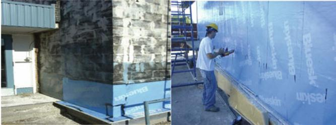
Fluid-applied air barrier installed over an existing exterior wall area and insulated with medium-density closed-cell spray polyurethane foam.
