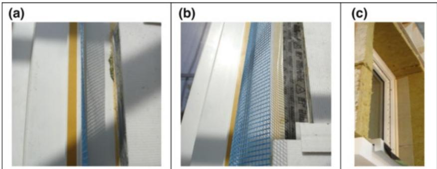
**Fig. E.13** Window/wall gap is sealed using mesh glued to the window frame from the outside using adhesive connector (c, d, e). Plaster is laid over the mesh and then painted over
