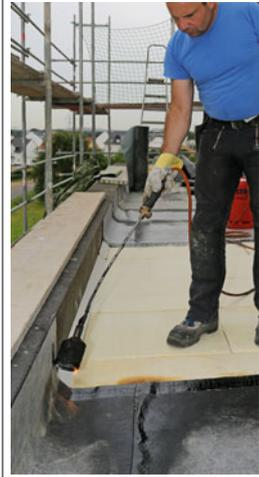
PUR rigid boards applied to a flat concrete roof in low-energy building and then covered by bitumen felt. Pictures: Puren ([www.puren.de](http://www.puren.de))
