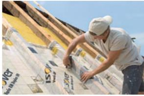
3b. Install the vapor retarder by passing it around the rafters and staple/tacker it without air gaps to the rafter
