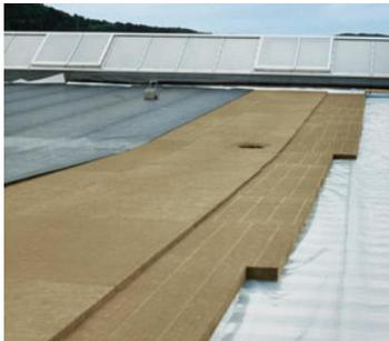
Flat roof insulation (stonewool) on a metal profile with waterproofing
