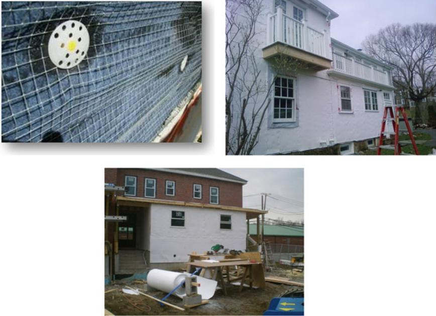
**Fig. C.18** Mechanically fixed with low thermal conductivity fixings (stainless steel and polymer). Finished with siding, brick slips, render, and mesh or cladding. Preserve building character due to thinner insulation profile
