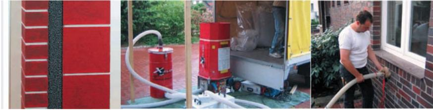
**Fig. 6.5** An example of a wall insulation, where insulation in the form of loose mineral wool is blown into the cavity. The experience with this kind of additional insulation is very good with low cost and almost no nuisance
