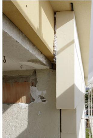
ETICS with rigid PUR boards being installed (by means of glue mortar) on solid wall during a building renovation. The boards are glued to the existing outside plaster by means of mineral glue mortar (point-strip application of the mortar to the rear face of the insulation boards), and later rendered. Source: puren ([www.puren.de](http://www.puren.de))
