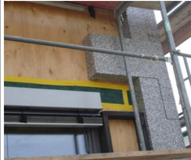
Example of a lamella mineral wool ETICS on a limestone wall (without need for mechanical fasteners, just 1 per m<sup>2</sup> as additional safeguard)
