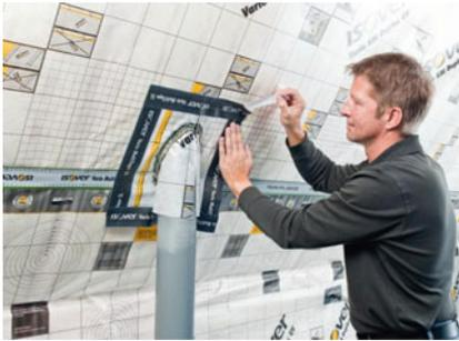
5. Adapt vapor barrier to pipes by using special tapes and glues. Follow the manufacturer's recommendations.
