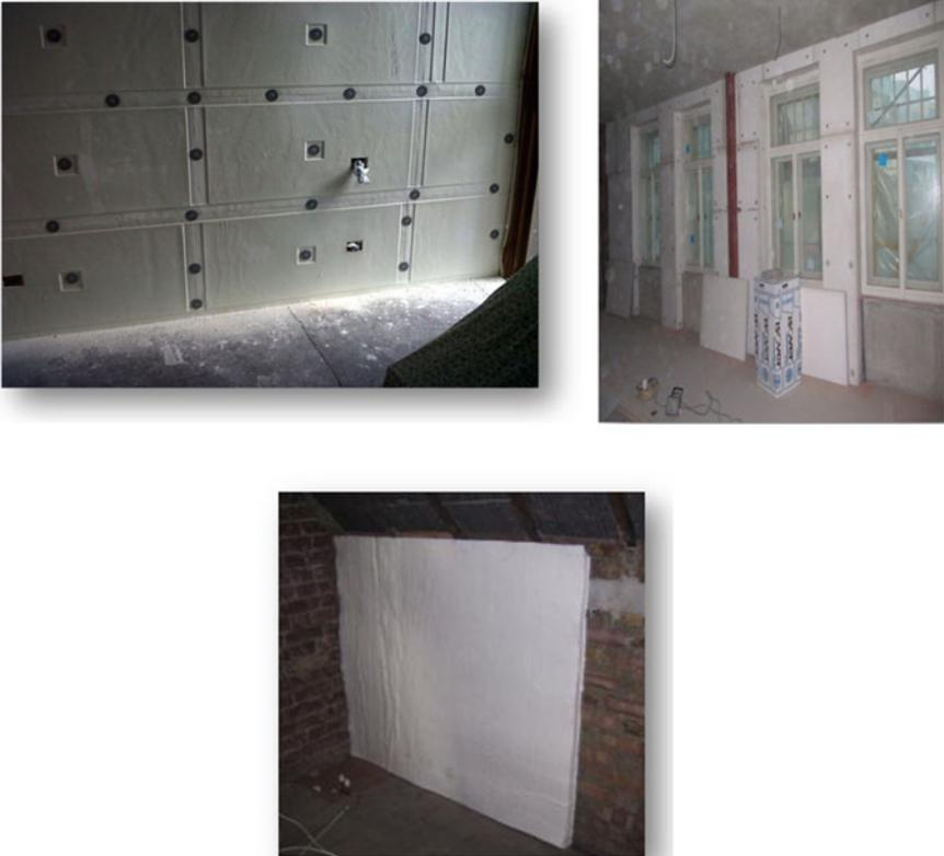
**Fig. C.17** Mechanical and adhesive fix to internal wall. Finish with wet plaster/lime or rigid facing board according to customer needs. Perform robust risk assessment to determine hygro-thermal impacts of IWI upgrade
