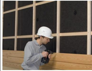
Ventilated façade with wooden supporting structure and wooden cladding profiles
