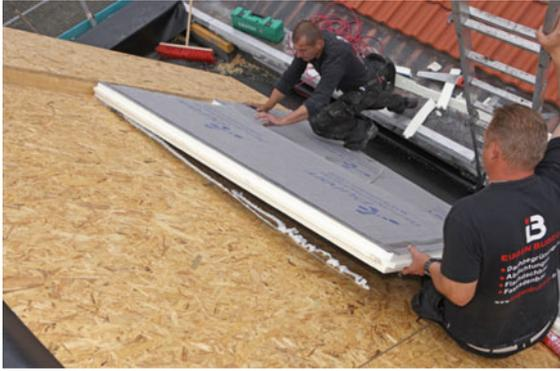
PUR rigid boards being installed on a lightweight roof and secured into place (during roof installation) by PUR spray foam stripes, beginning with the lowest board
