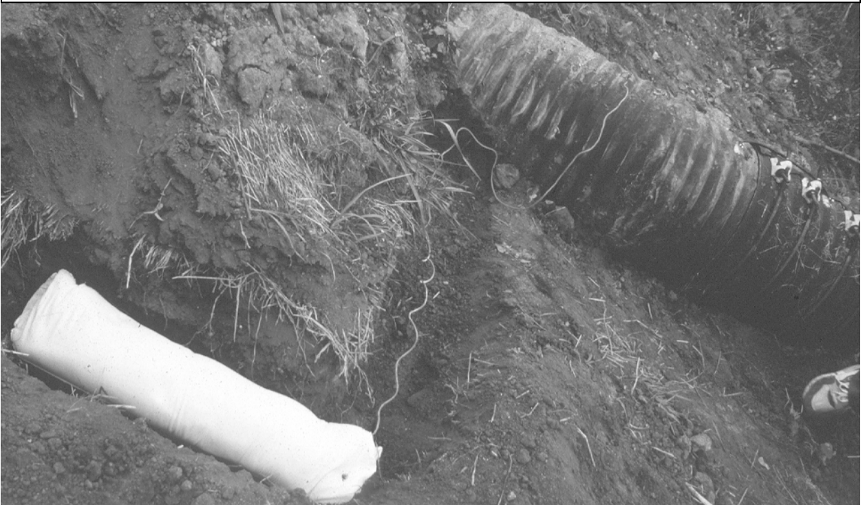
Figure 6. Installing Horizontal Mg Anode Next to Pipe
