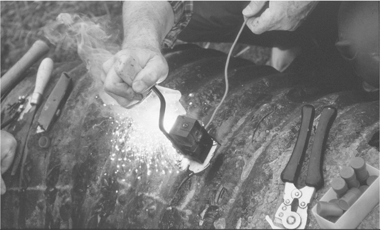
Figure 7. Thermite Brazing (Cadwelding) Mg Anode Lead Wire to Pipe
