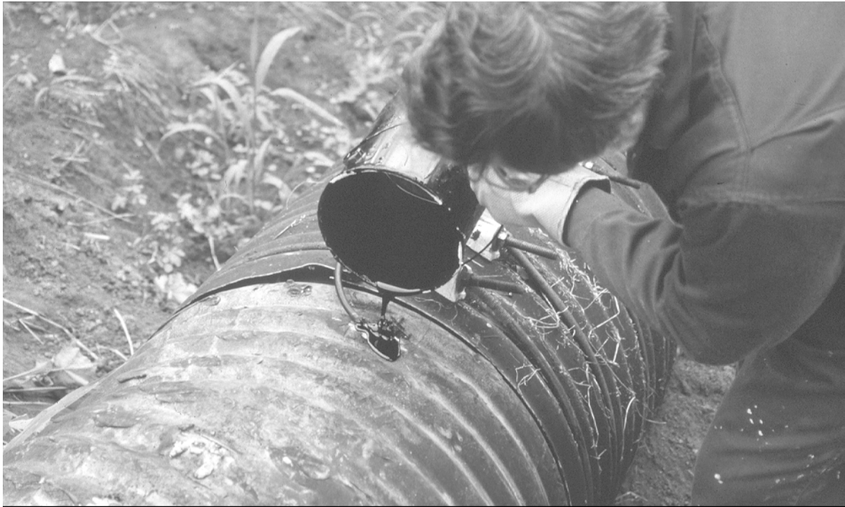
Figure 9. Pouring Waterproofing Compound over Completed Thermite Connection
