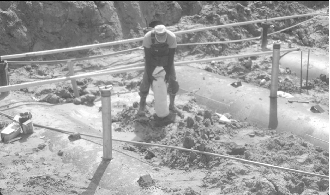
Figure 6. Installing Horizontal Mg Anode Next to Pipe
