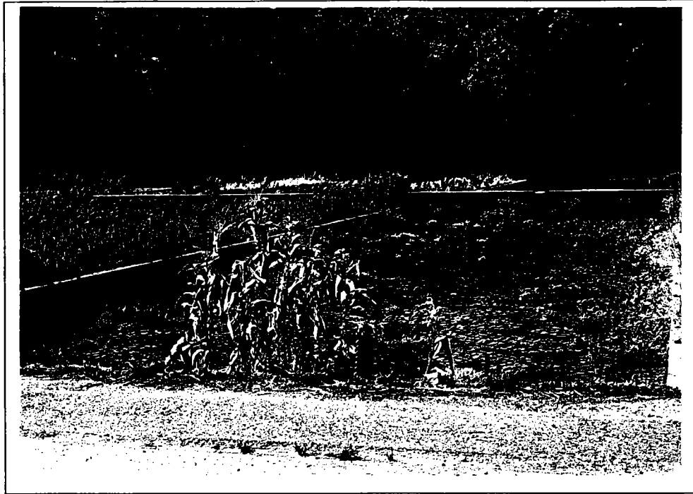
CORN AND WEEDS GROWING IN SLUDGE DRYING BEDS
