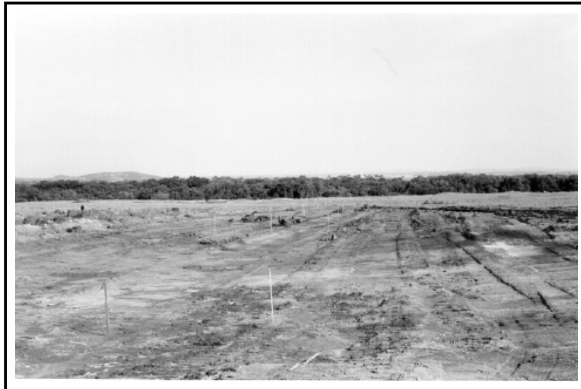
Figure A-26. Earthwork and grading.
