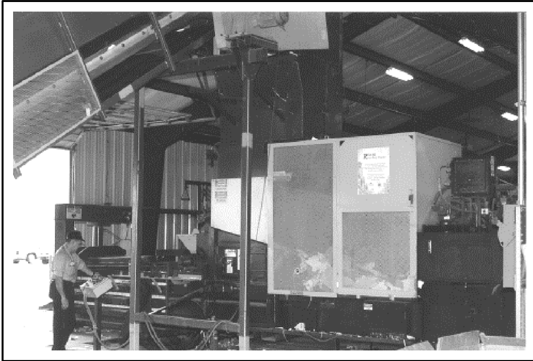
Figure A-3. Paper baler at Fort Sill.
