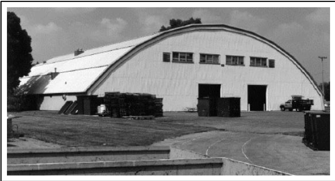
Figure A-1. Recycling building at Fort Riley.
