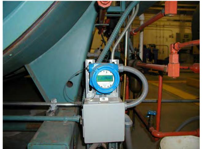
Figure 4. Oil meter on a DACH boiler.
