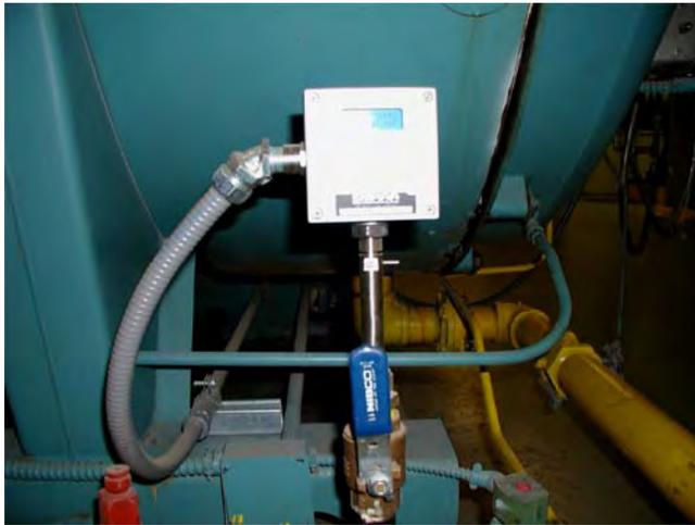
Figure 3. Gas meter on a DACH boiler.
