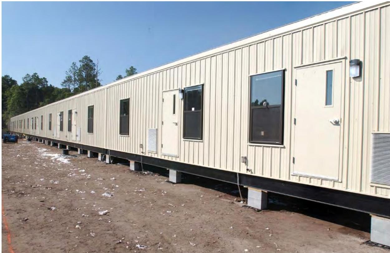
Figure A-4. Joined modular units awaiting exterior work.
