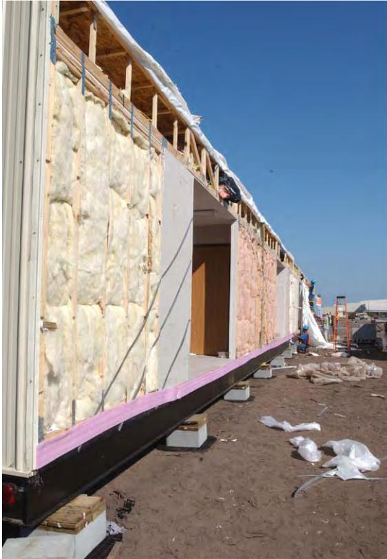
Figure A-3. Modular units being prepared to be joined together.
