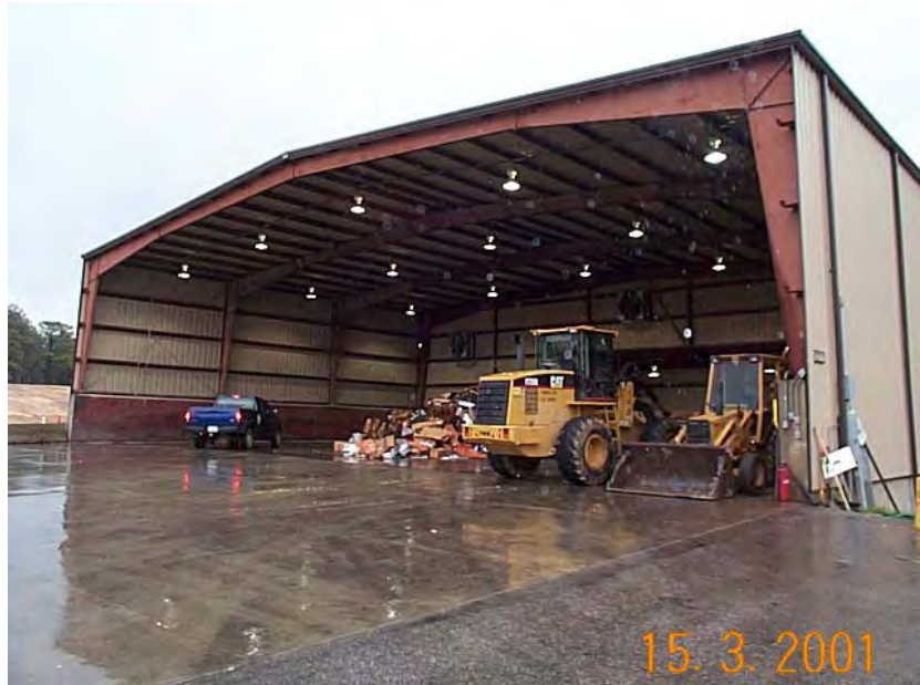
Figure A-1. Transfer station.
