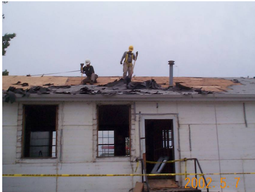
Figure 1. Removal of asphalt shingles during deconstruction of a WWII Army barracks.
