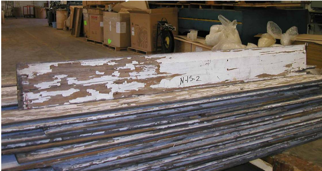
Figure 8. Salvaged wood siding containing lead-based paint.
