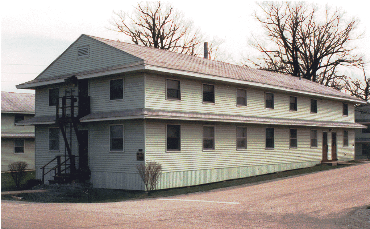
Figure 6. Vinyl-sided two-story Army barracks.
