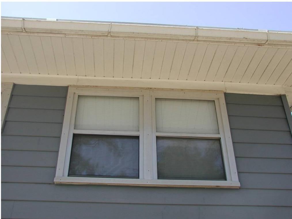
Figure B-4. Typical aluminum window of an eight-unit family housing building.
