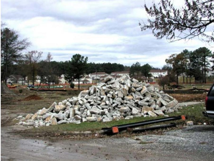
Figure A-1. Concrete recycling at Fort Bragg.
