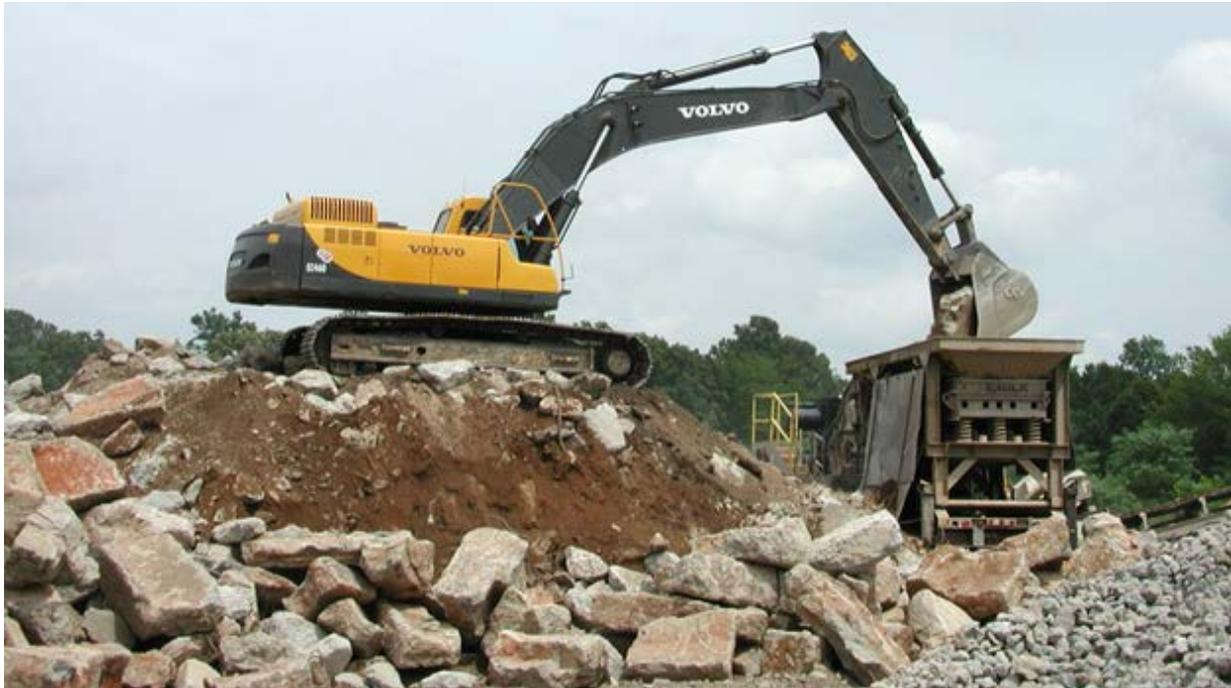
**Figure C-1. Concrete recycling with on-site crusher.**
