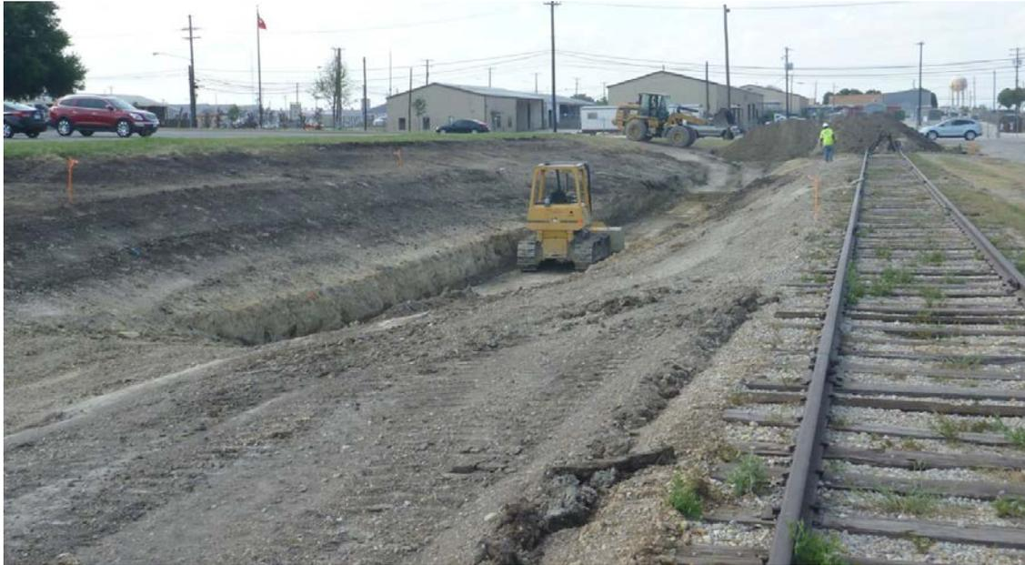
Figure B-3. Bioswale trench excavation.
