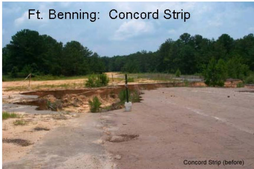
**Figure A-3. Lack of on-time repairs resulted in localized erosion and NPS pollution at Fort Benning.**
