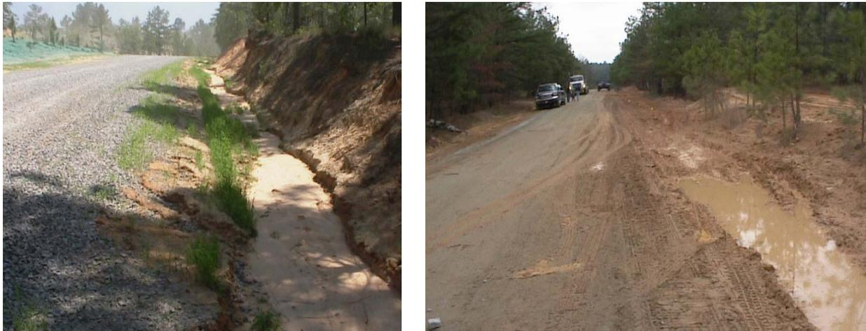
**Figure A-2. Road shoulder erosion is among the most significant contributor of NPS pollution at Army installations.**
