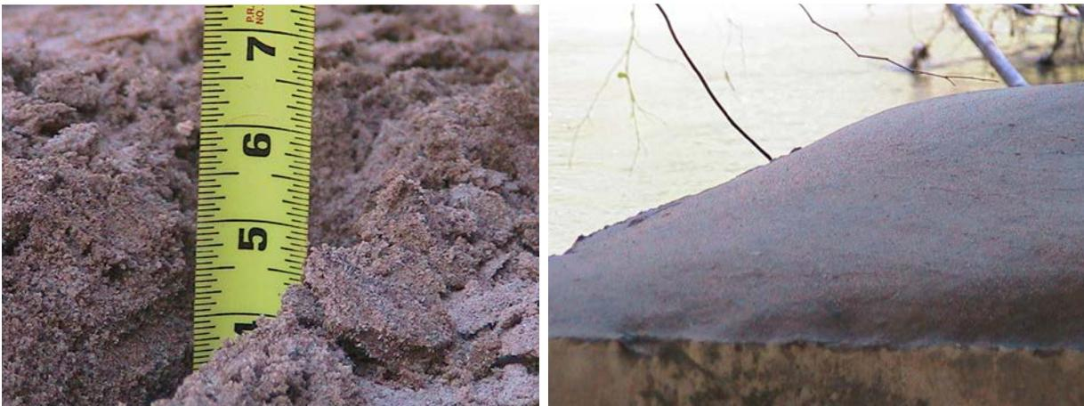
Figure E-1. At Randall Creek, 2nd Armored Division Road, one storm dumped 7 in. of sediment on a pier almost 4 ft above streambed.
