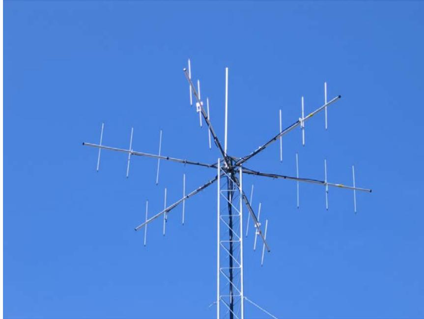
**Figure A-4. An example of the antenna array used with the ARU system. An array with six antennas is affixed on top of a tower and aligned every 60 degrees to fully cover the surrounding landscape.**
