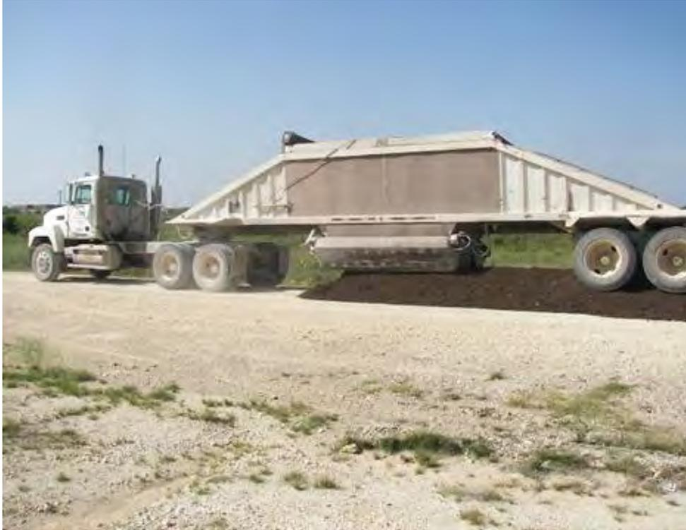
**Figure A-5. Belly-dump applying asphalt mix to tank trail.**
