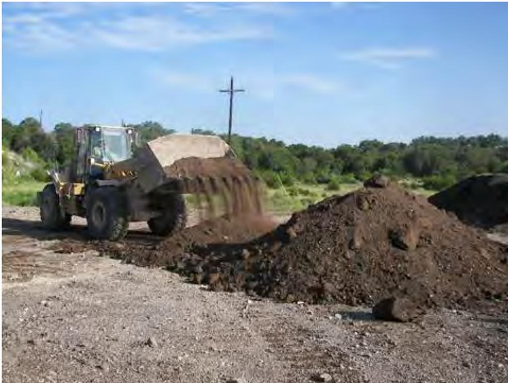
**Figure A-4. Front loader mixing asphalt shingles and recycled roadway asphalt.**
