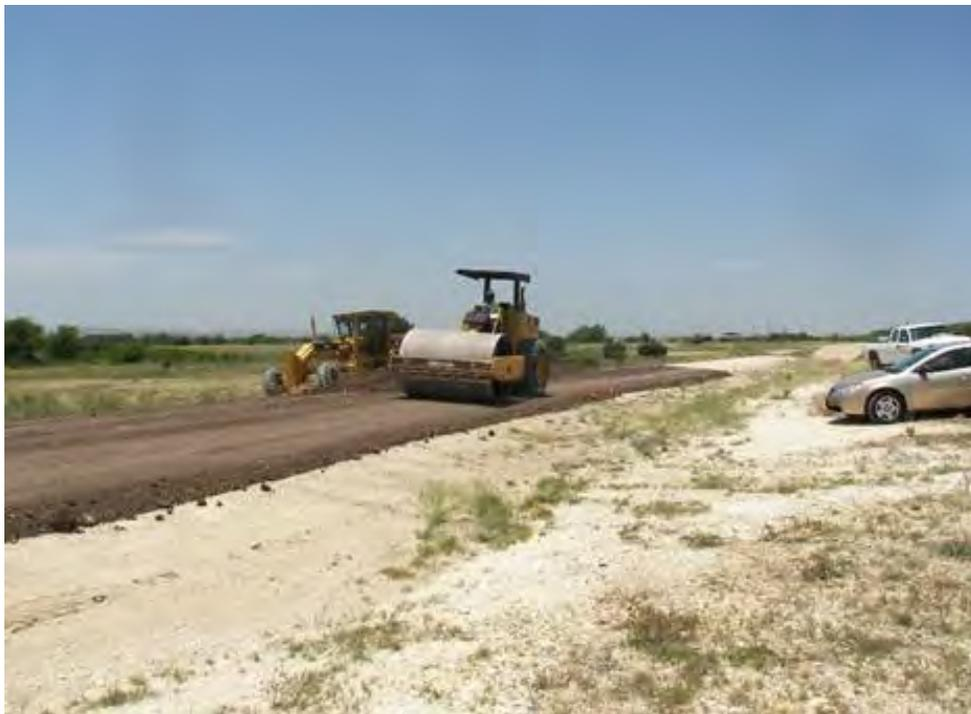
**Figure A-6. Equipment spreading and compacting asphalt mixture.**
