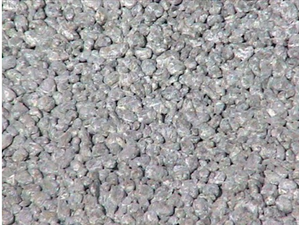
Figure A-4. The Ecocrete porous concrete finished surface.
