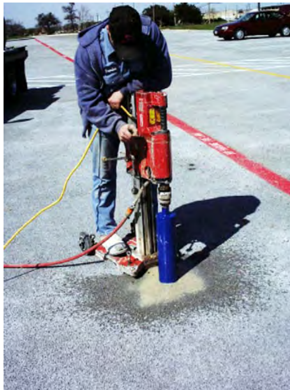
Figure A-5. Hole saw used for drilling a sample port.
