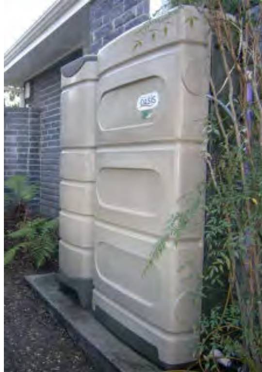
Figure 9. Example of Australian technology for graywater storage.
