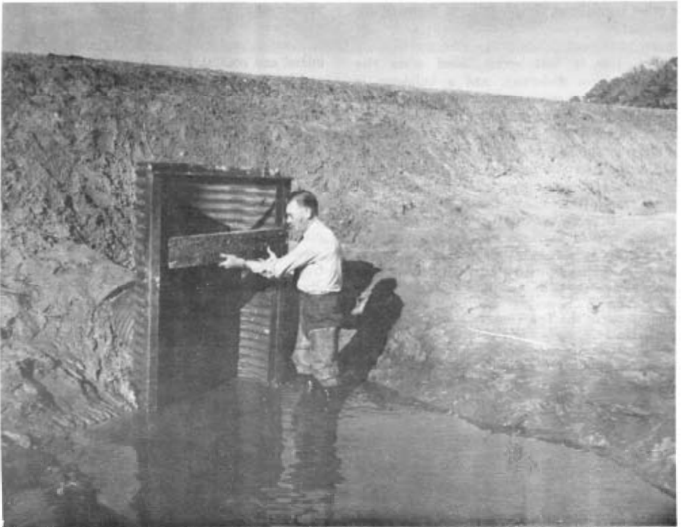
Figure 6-3. A flashboard riser for controlling water levels.
