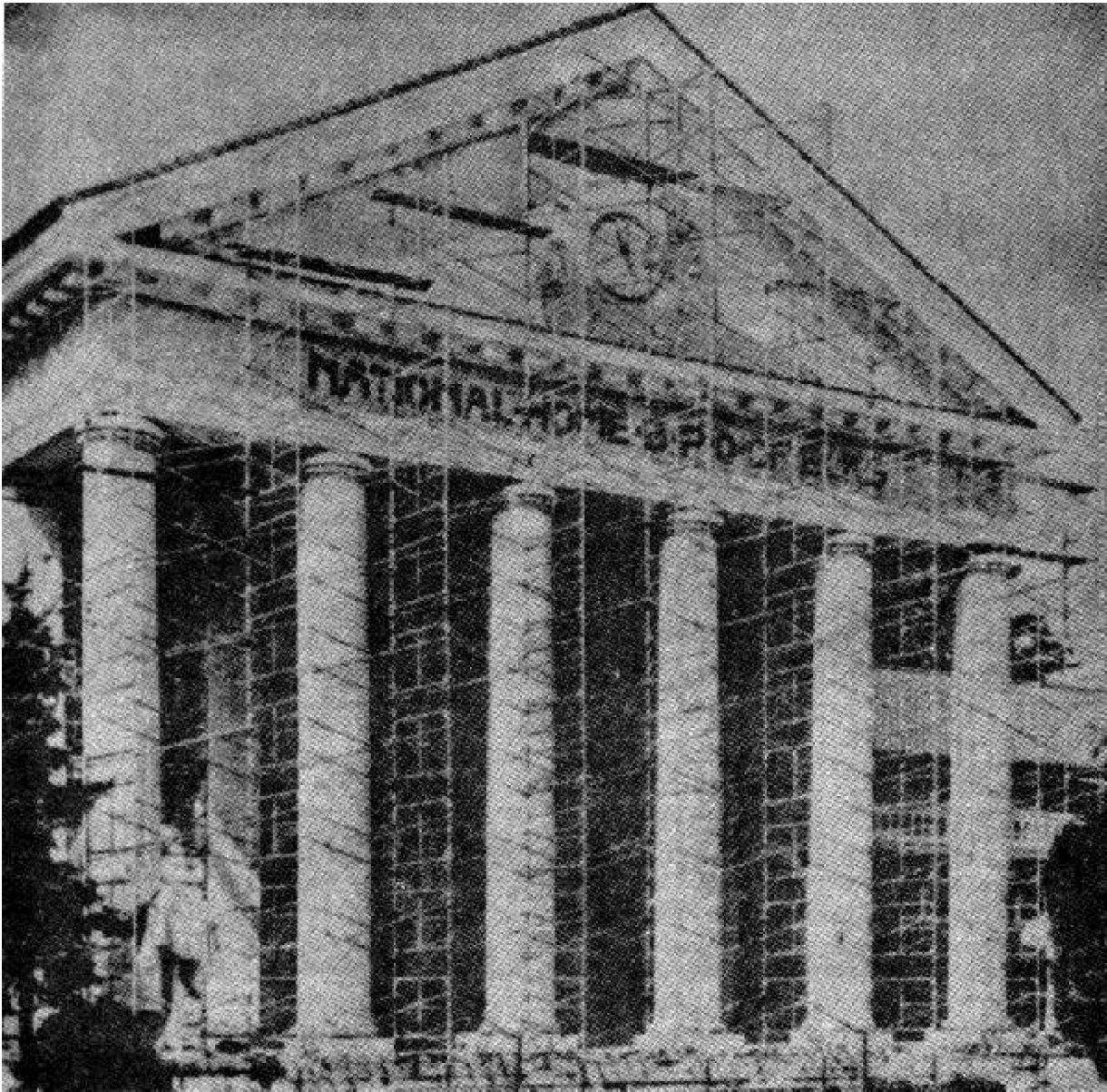
FIGURE 3-19 Pipe Scaffolding
