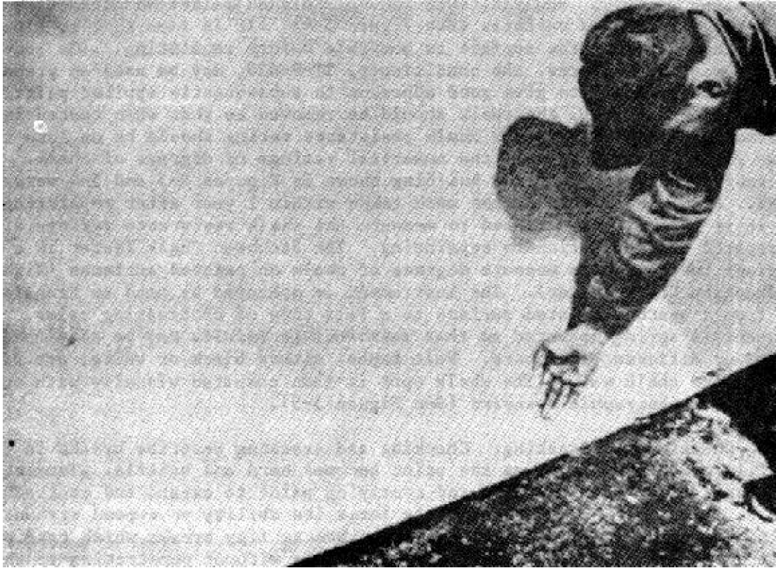
FIGURE 5-2a Severe Chalking
