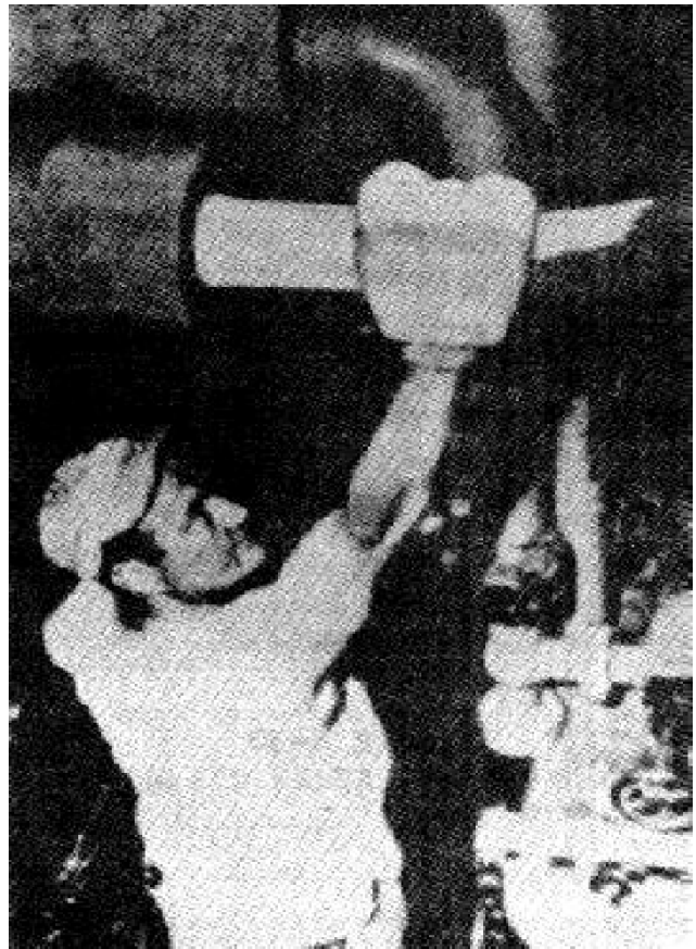
FIGURE 4-47 Paint Mitt In Use
